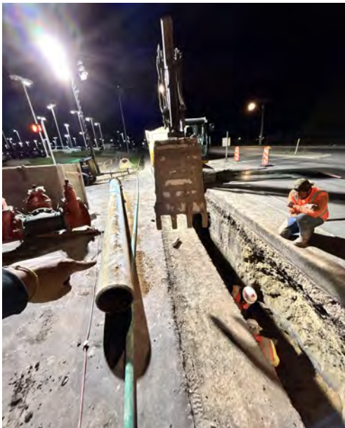
Installing pipeline at 700 West 3300 South
