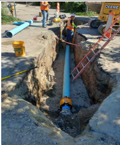
Installing the last stretch of PVC pipe on Empire Ave
