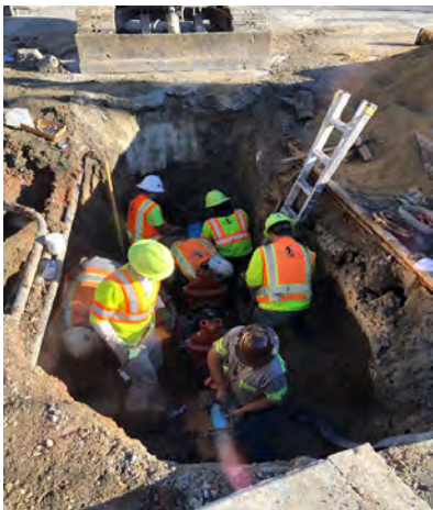
New valving at 4500 South 700 East to restore water service
