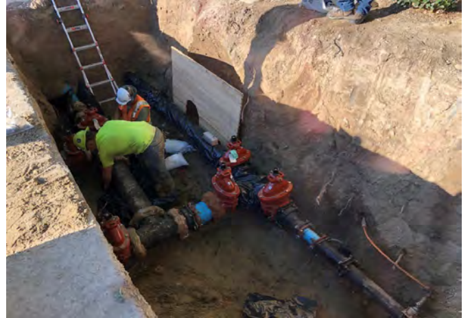
New valve clusters replacing the old vault at 4600 South 700 East
