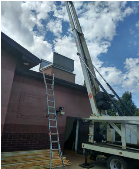
Well rig on-site for final development work
