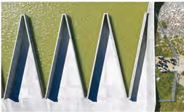
The DMAD Reservoir spillway is looked over as the Millard County Farm Bureau hosts a tour of alfalfa farms, water improvements and a dairy to showcase local agriculture in Delta on Sept. 6. The dam is the largest accordion-style variety in the West.
