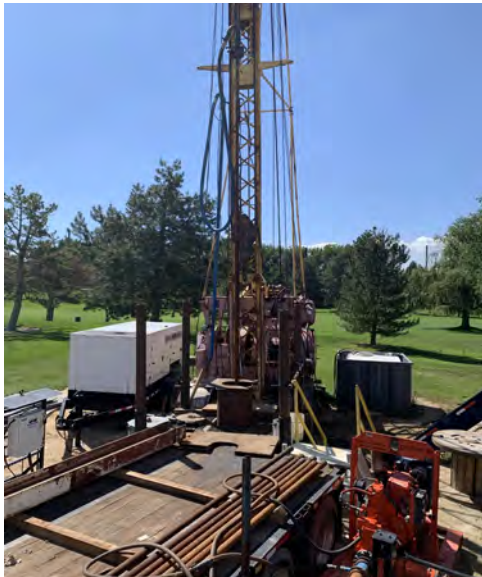
Drill rig performing chemical treatment
