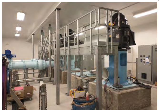
New pump, motor, and access platform installed in pump station
