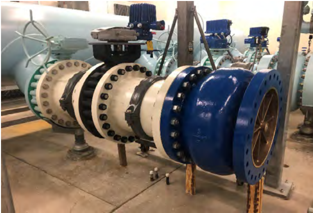
Installing 24-inch discharge piping
