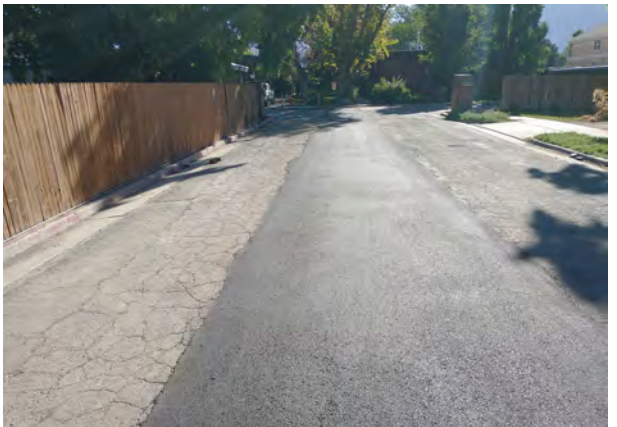
New asphalt over completed line on 3720 South
