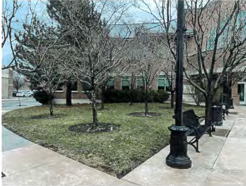
South Jordan City Hall Before
