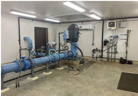
DW7 Well Motor awaiting final installation
