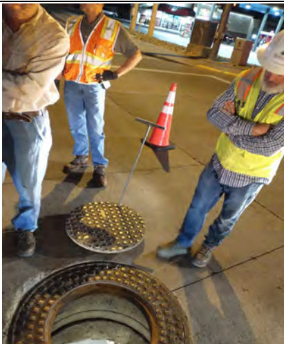
Accessing 700 East 11400 South vault early to avoid heavy traffic
