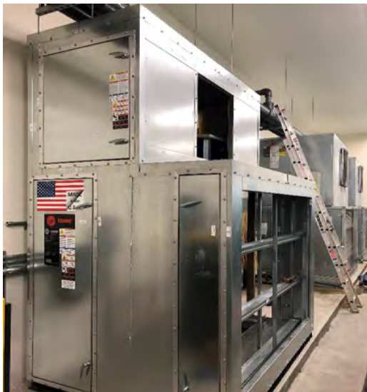
Assembling new air handling unit
