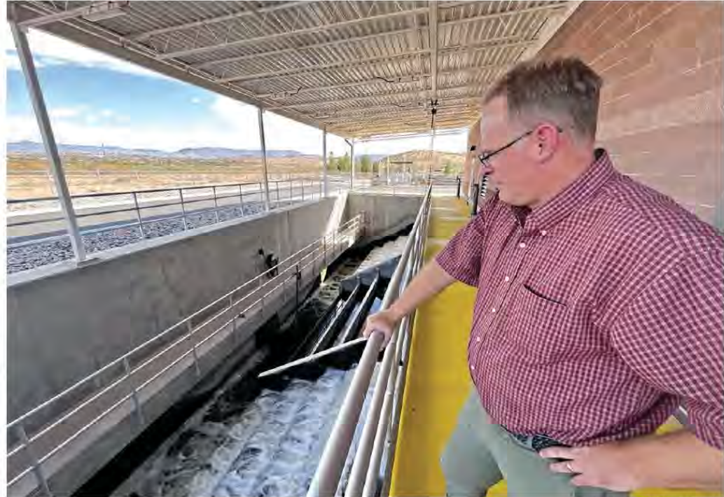
St. George Water Services Director Scott Taylor watches as treated sewage leaves the city's plant and flows downstream toward Lake Mead. The city is finalizing plans for a new reservoir that will allow it to store more recycled wastewater for future use.
