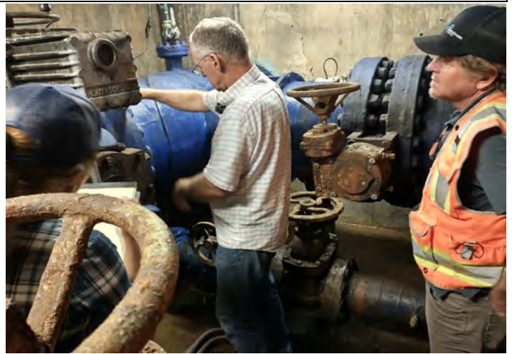
Evaluating the valves and piping in the 200 East 11400 South vault
