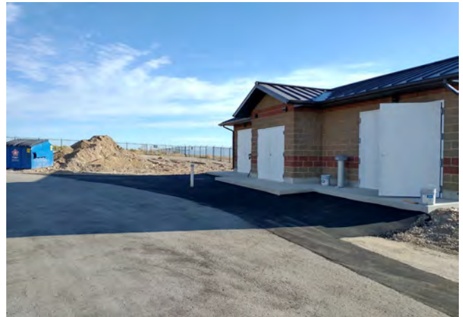
New chemical feed building with new asphalt
