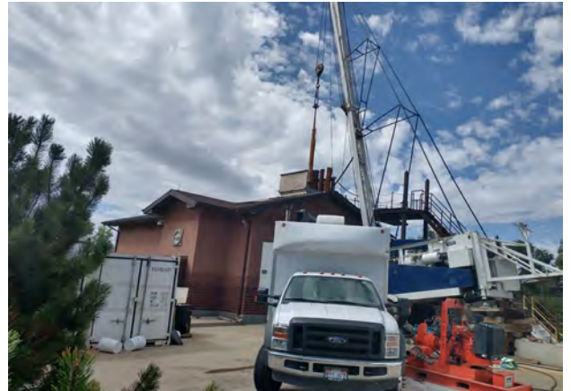
Well rig on-site for final development work
