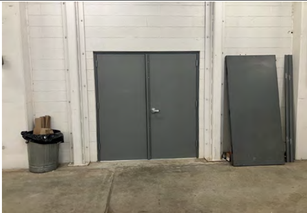
New sound doors installed
