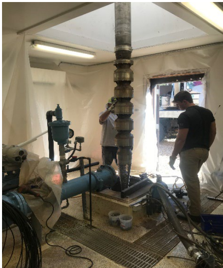
Pump Re-installation
