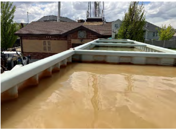
Silt being removed from the well during well-redevelopment
