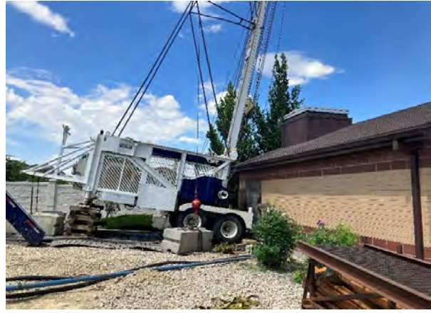
Well Redevelopment Machine
