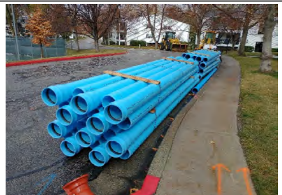
New PVC pipeline ready to be installed
