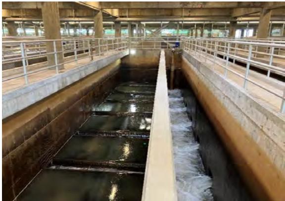
Filter backwash launders will be raised to accommodate deeper filter media
