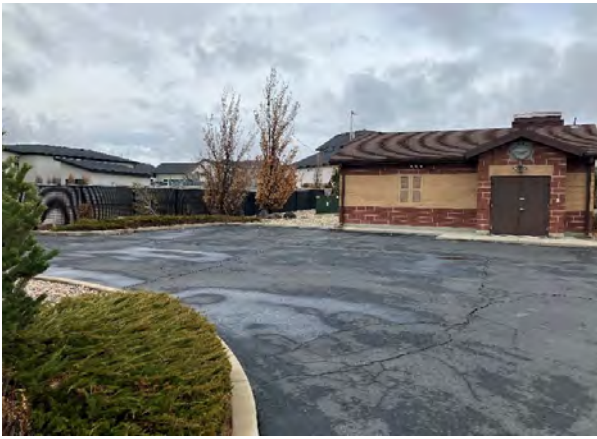
DW7 Well Pump House
