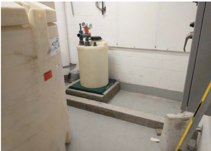
New concrete curb and pedestal for day tank
