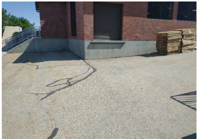
Existing forklift loading area to receive concrete pad in this project
