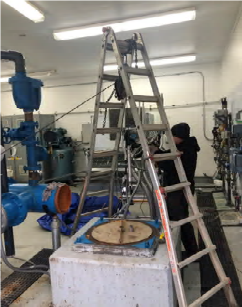
Setting up rigging to video the well
