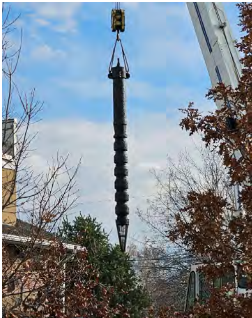
Pulling existing pump from the well
