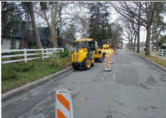
Contractor equipment mobilized at Old Farm
