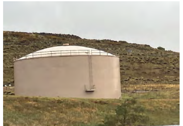
A second backwash tank will be constructed with this project to provide redundancy
