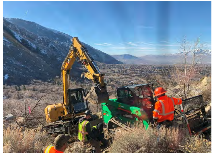
Mobilizing construction and inspection equipment near the Bell Canyon Reservoir.
