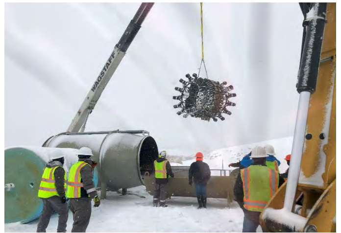
Loading the inspection into the JA-1. This tool is slowly pulled through the pipeline to measure wall thickness. It can detect anomalies as small as .25 square inches
