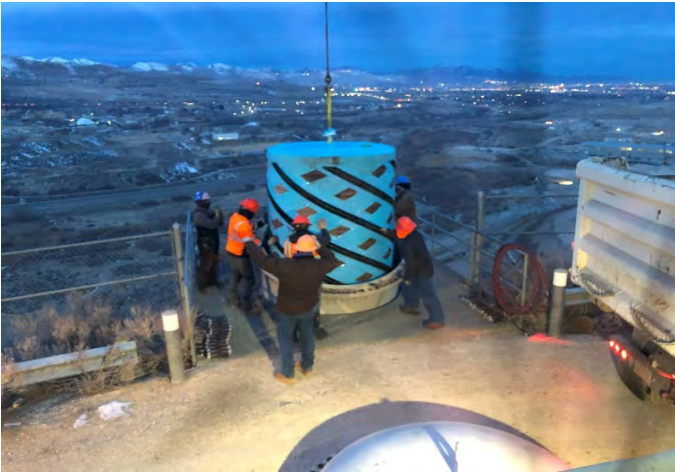
Cleaning JA-1 prior to the condition assessment inspection tool
