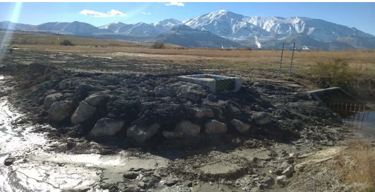
Pipeline discharge structure
