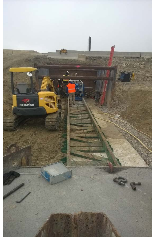
Jack & bore under the freeway
