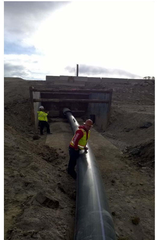
Pipeline being pulled through casing
