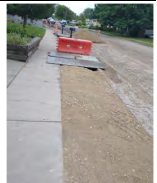
Park strips and drive approaches partially restored after installing pipeline
