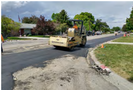
Contractor laying asphalt in Murray
