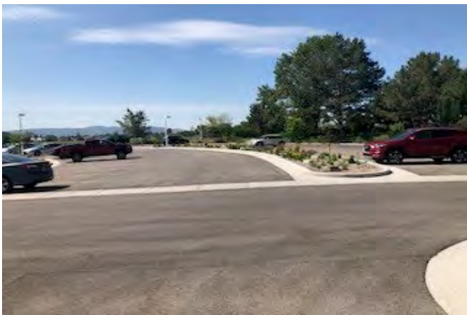
South parking area of Admin Building
