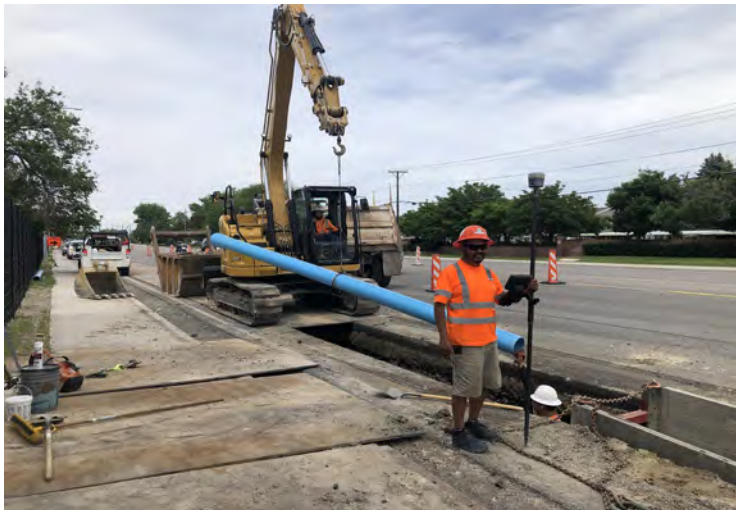
District staff collecting GIS data on new pipeline
