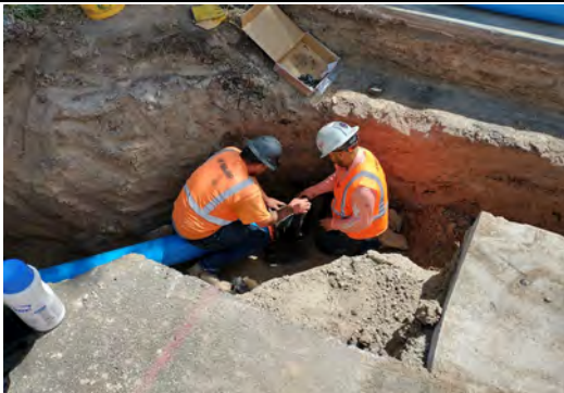
Installing a new bend on the new PVC pipeline
