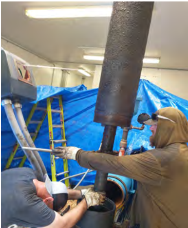
Contractor pulling the pump column from the well
