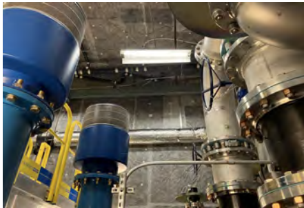
Installed insulation over welding room blower duct
