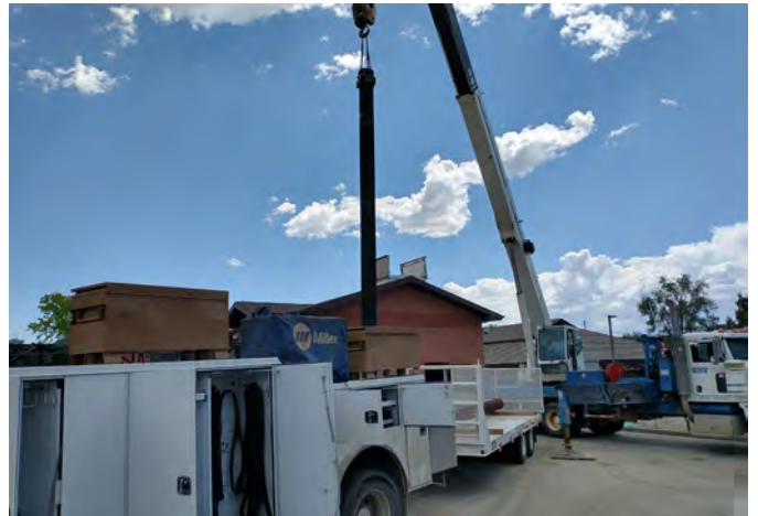
Section of pump column being set on trailer
