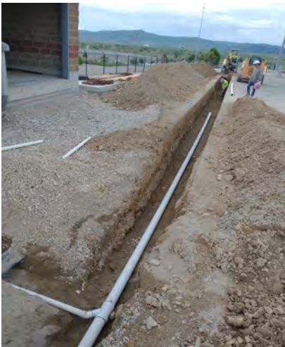
Contractor installing drain piping for new building
