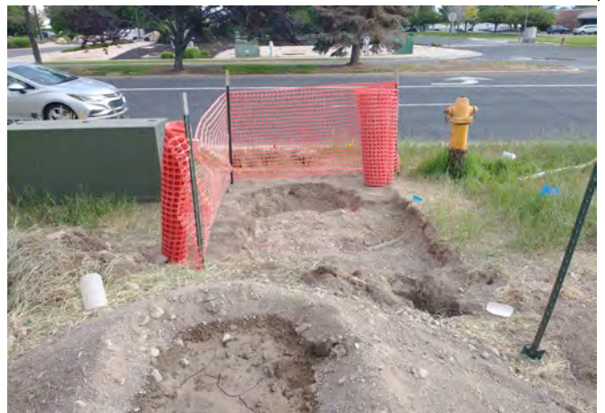
Excavation to install transformer pad
