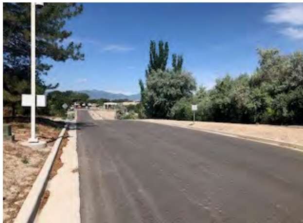
Beckstead Lane roadway improvements
