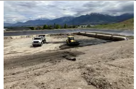
District staff removing dried sludge from the new concrete-lined backwash basin
