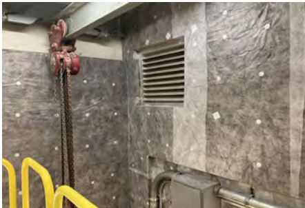
Installed acoustical insulation
