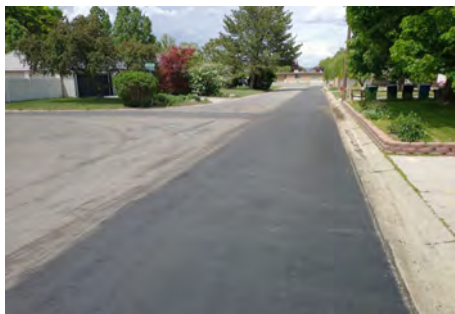
New asphalt laid over the new pipelines
