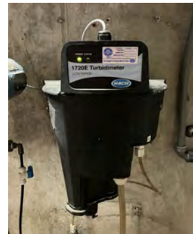
Settled water turbidimeter to be upgraded with this project
