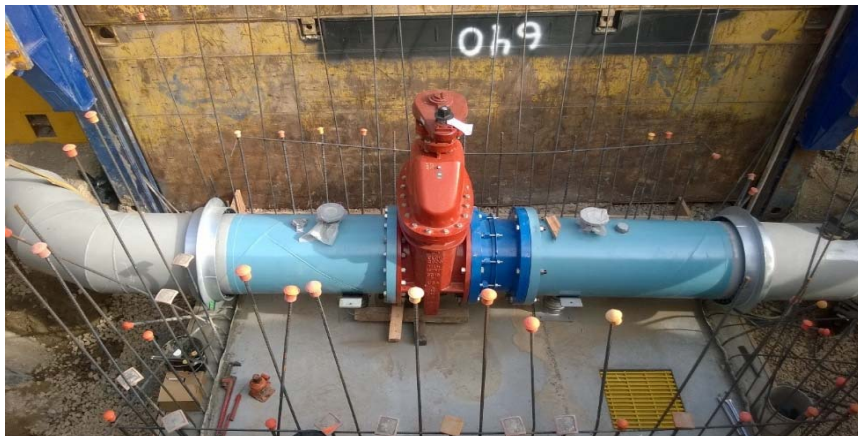
Main Street 4500 South new isolation valve and rebar installation
