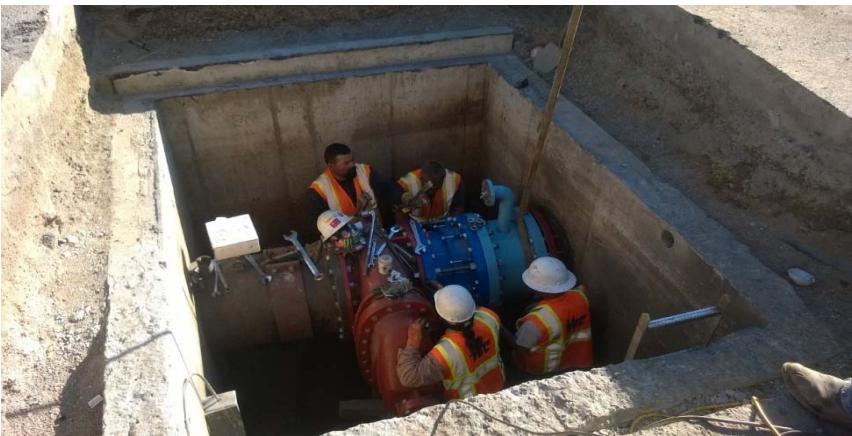
900 East 4500 South installation of new main line valve
