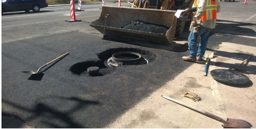
900 East 4500 South repair of roadway above new concrete deck lid
