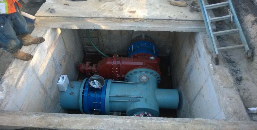
Murray Holladay Road 1300 East new piping being installed
