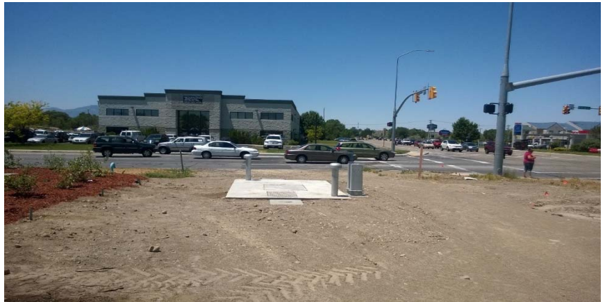
500 West 4500 South finished PRV vault
