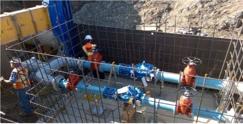
500 West 4500 South PRV vault rebar installation
