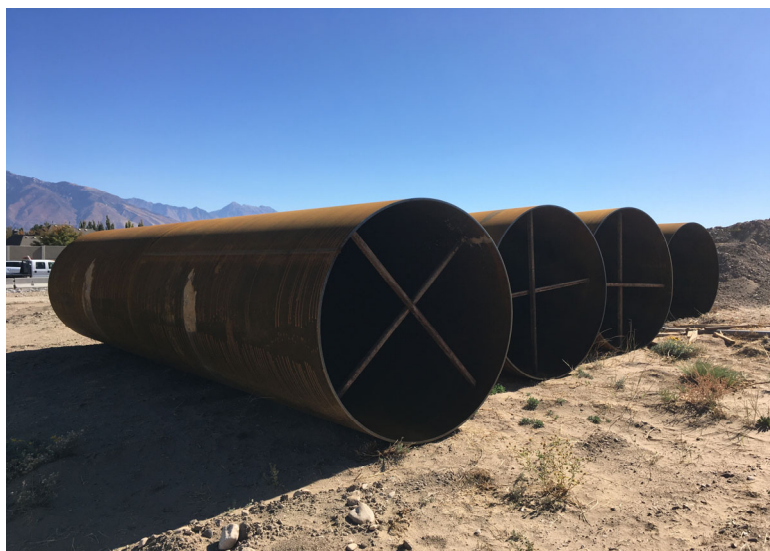
60" casing prior to installation
