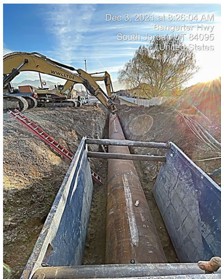
Installation of the 60" casing through the JA-2 easement
