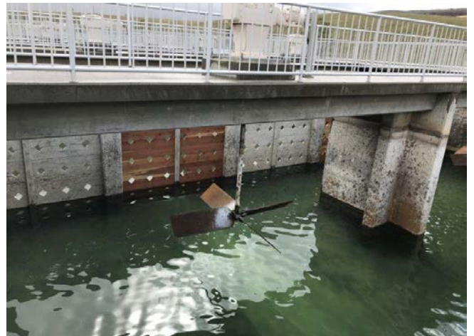
Basin testing after completion of work.
