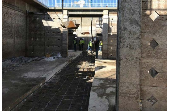
Preparing for first concrete placement.
