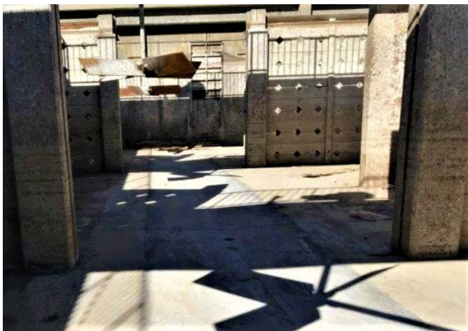
Completed basin trench.
