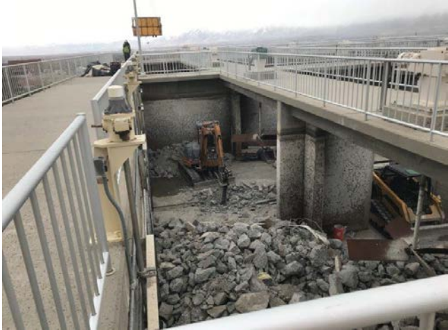
Demolition of old concrete trenches.
