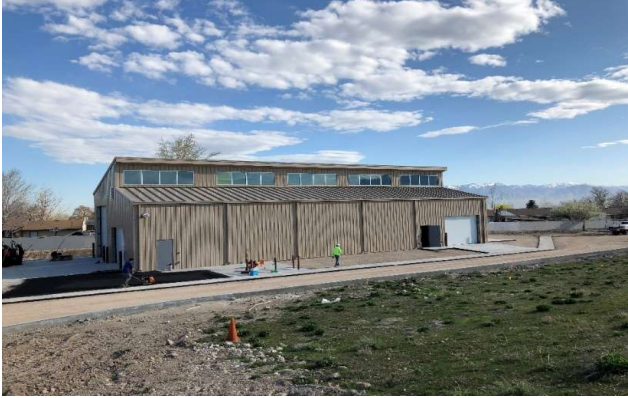
South View of Building
