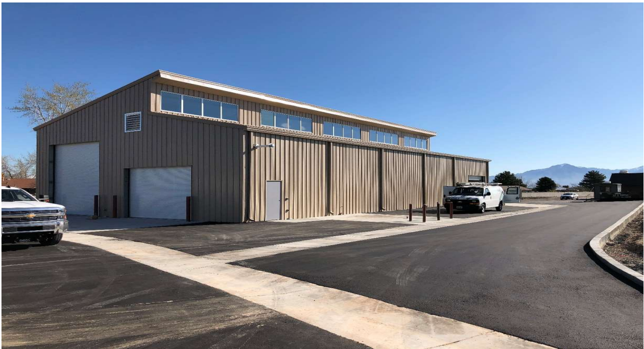
Southwest of Completed Building
