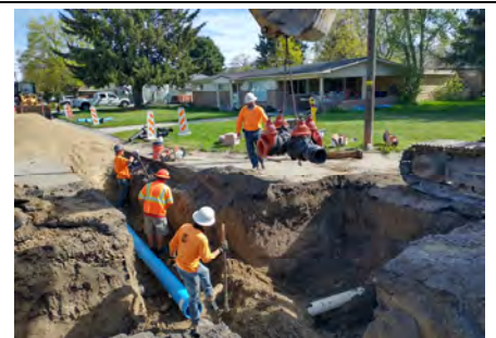
Installing a 4-valve cross at an intersection
