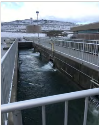
JWTP Basin 1 in operation
