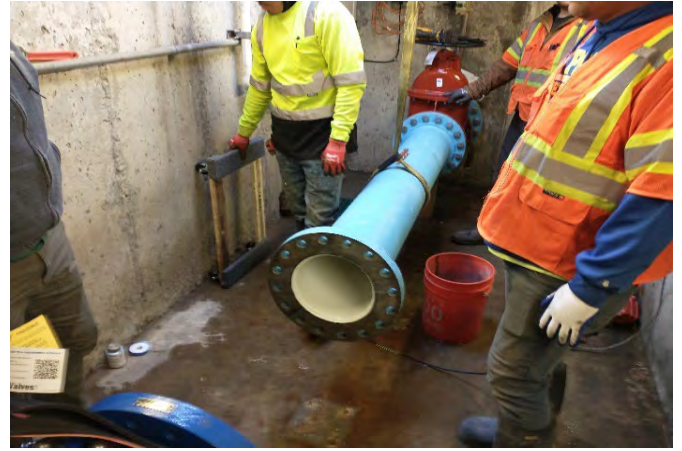
Installing new pipe in vault
