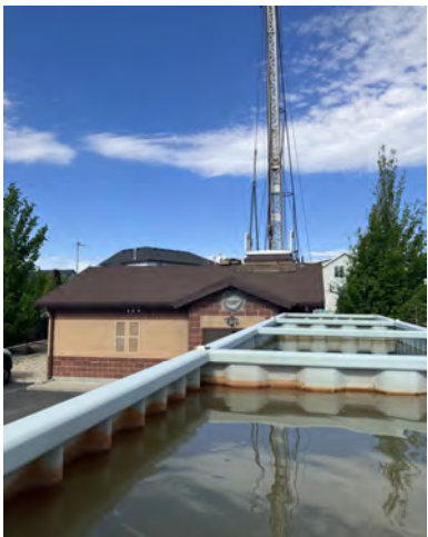
Ongoing well development work at DW7
