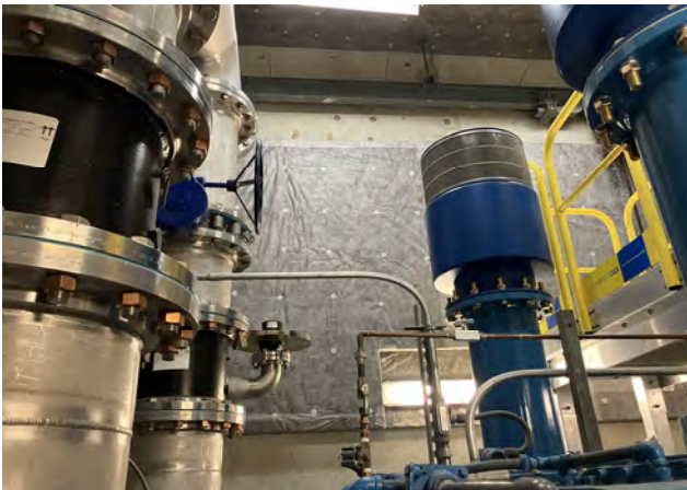
Acoustical foam installed in JWTP Blower Room
