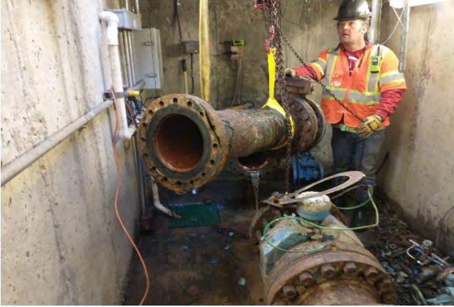
Removing the old corroded pipe
