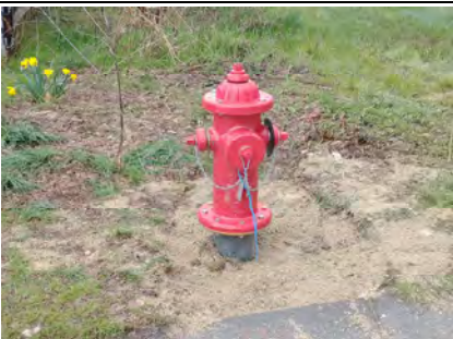
A new hydrant installed in the project area
