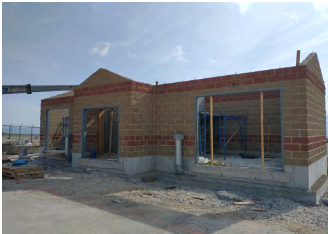
New chemical feed building being constructed
