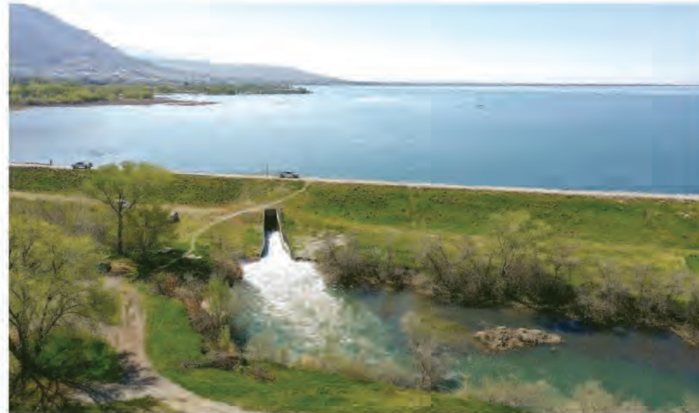
The Willard Bay spillway gates are opened for flood mitigation in Box Elder County on Thursday.
