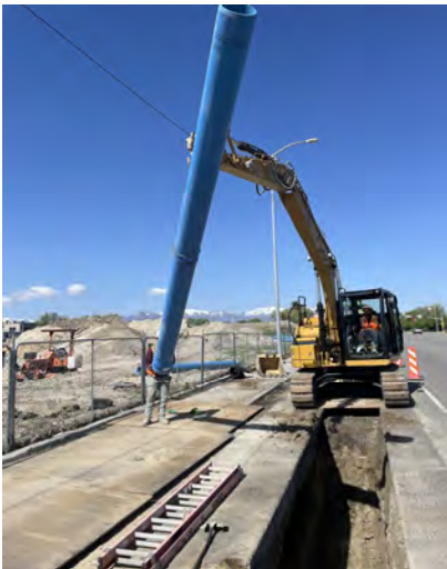
Installing 12-inch PVC pipeline
