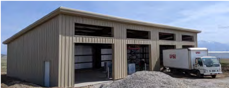
Building's Southwest view
