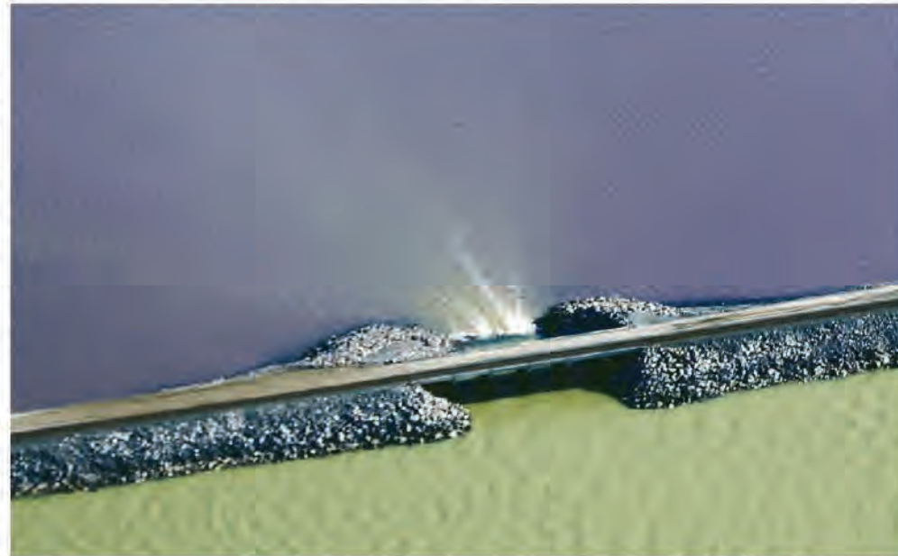
The railroad causeway is breached on the Great Salt Lake as photographed on Wednesday.
