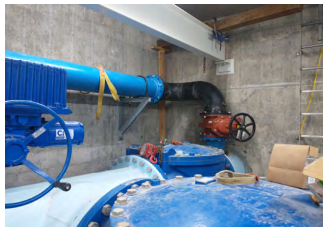
New pipeline tied into existing vault
