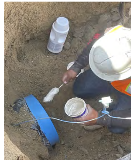
Applying lubricant to pipe gasket
