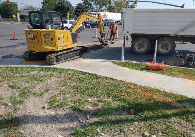
Trenching in Roadway by vault.
