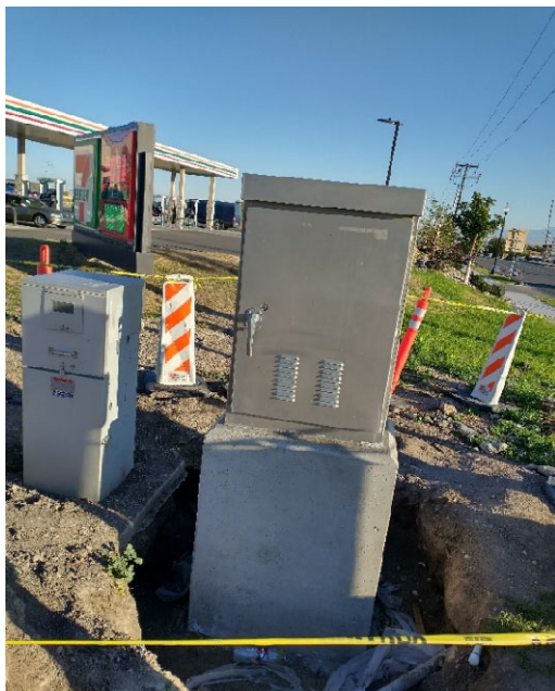
New RTU pedestal outside vault.
