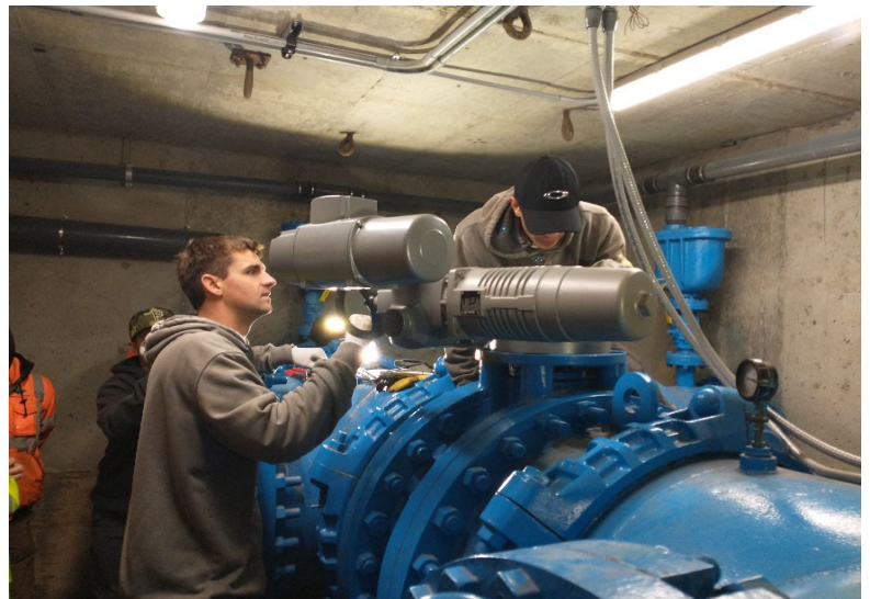
Installing new valve actuator.
