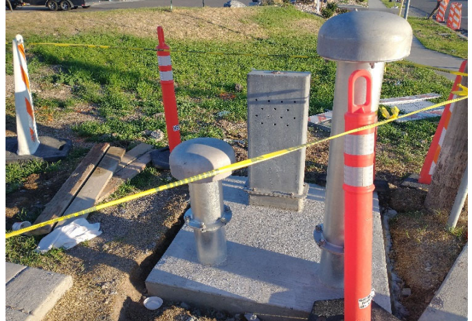
New concrete pad for vents.
