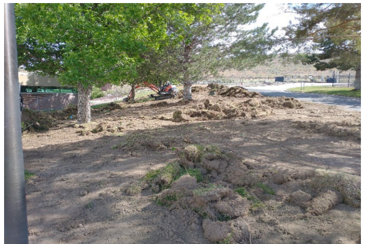
South Area of Project being grubbed
