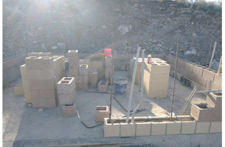
Constructing building walls at Rosecrest
