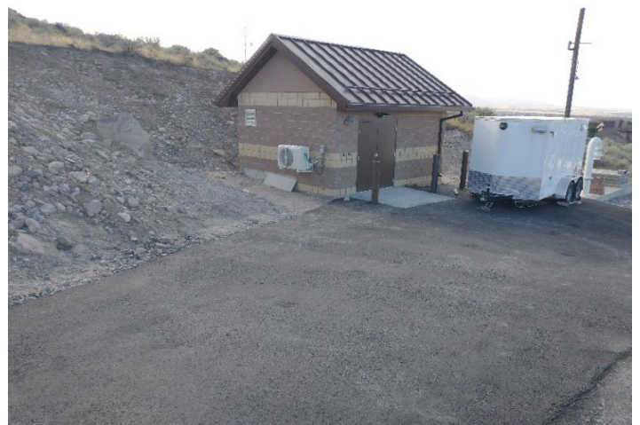
Completed Rosecrest building
