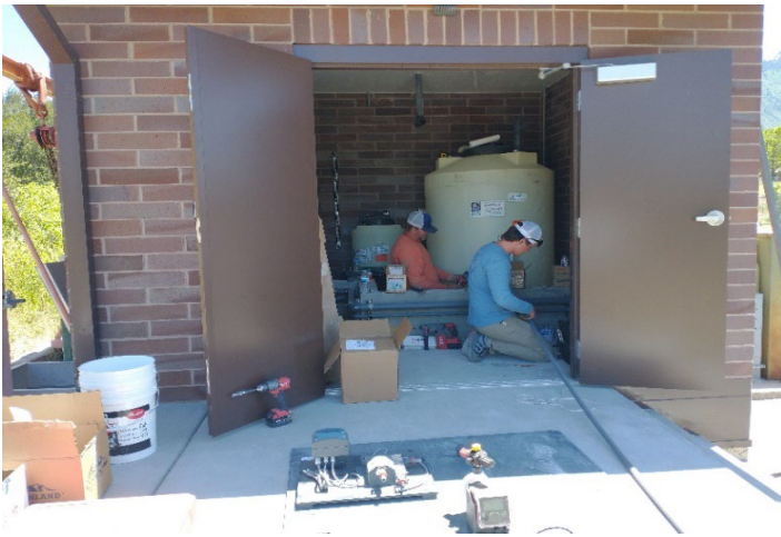
Installing tanks and piping at 9800 S 2300 E
