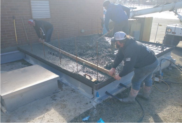
Laying building foundation at 9800 S 2300 E
