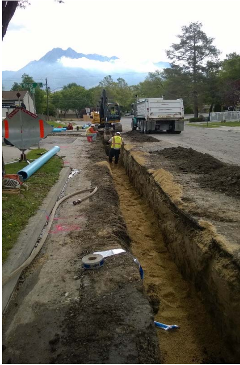
Laying pipe along Chevy Chase Drive
