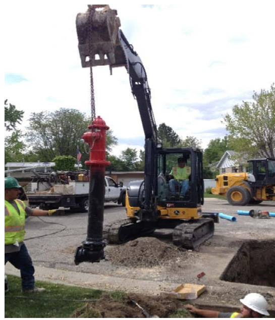
Installation of a new hydrant on
