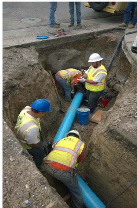
Chevy Chase Drive tie-in to Revere Drive
