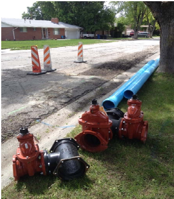
Valving to be installed on Chevy Chase Drive
