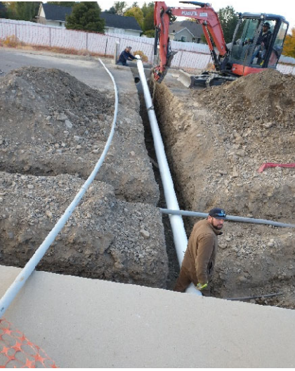
Laying blowoff Piping at Cedar Hills Location
