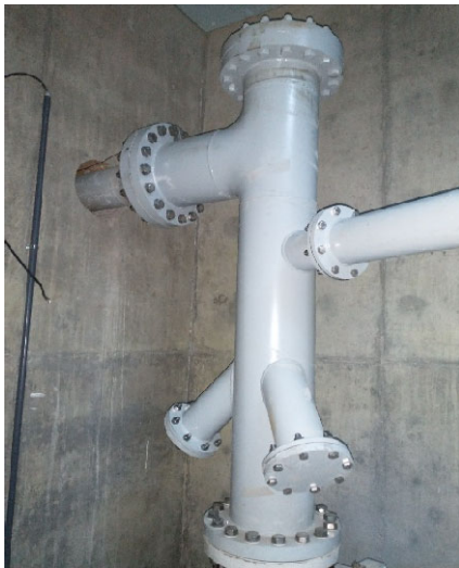
New Vault Piping at Cedar Hills Location
