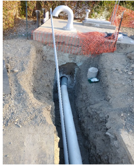
Laying blowoff Piping at Pleasant Grove Location
