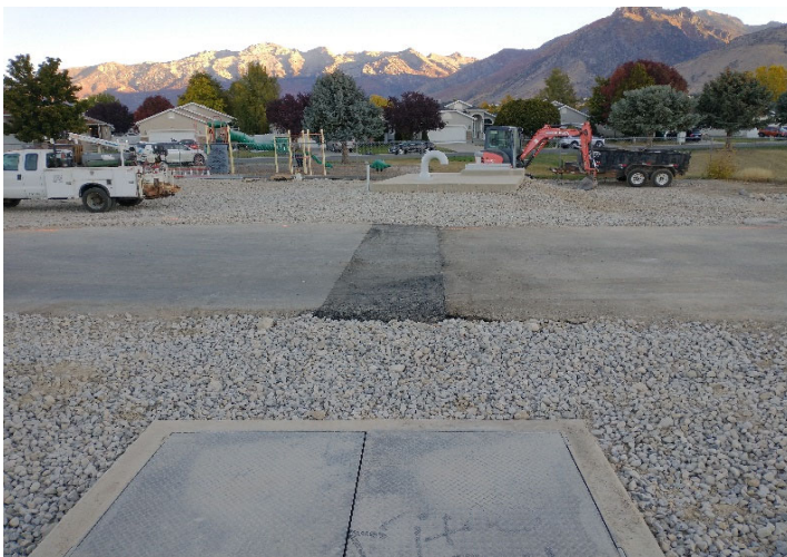
Final surface restoration at Cedar Hills Location
