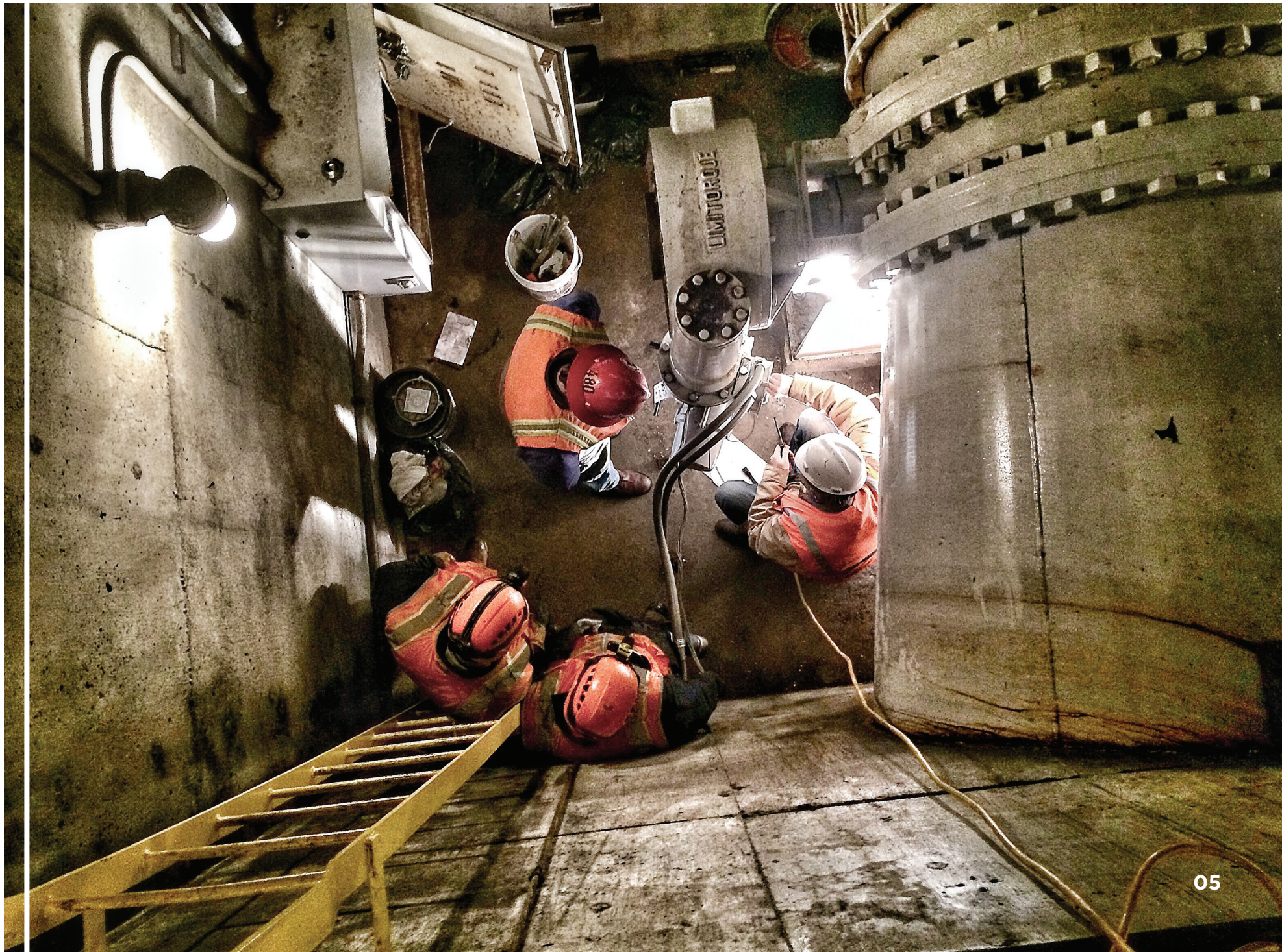
Crews install an actuator on a valve. Photo by Alex Mitchell.
