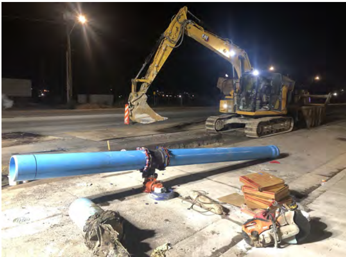
Preparing to install 6-inch auxiliary valve for fire hydrant
