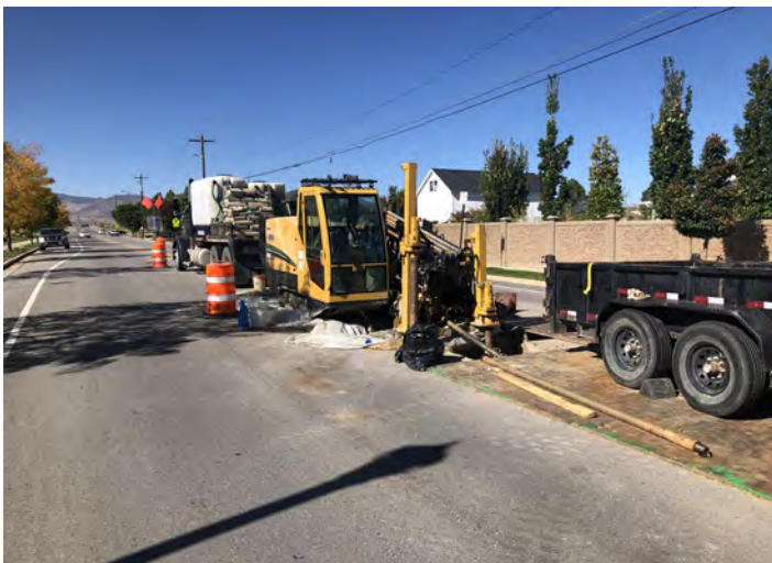
Direction drill rig to install AC mitigation cable
