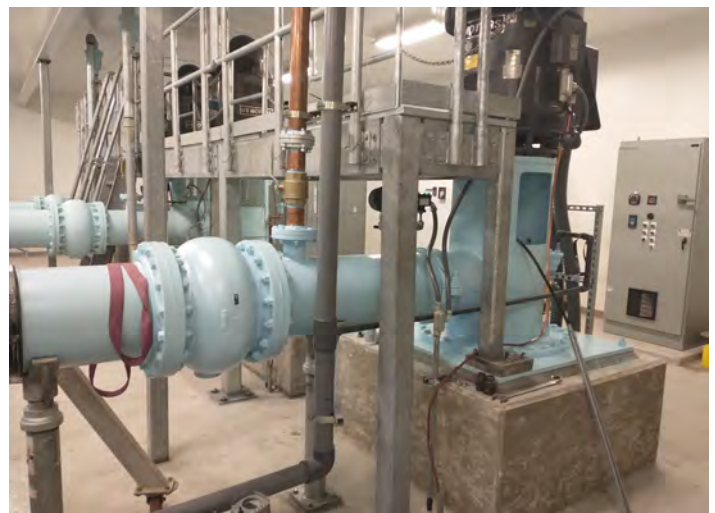
The new pump, motor, and piping installed and coated
