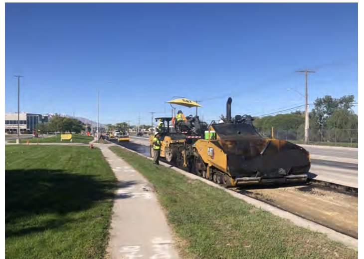
Placing asphalt along 3300 South
