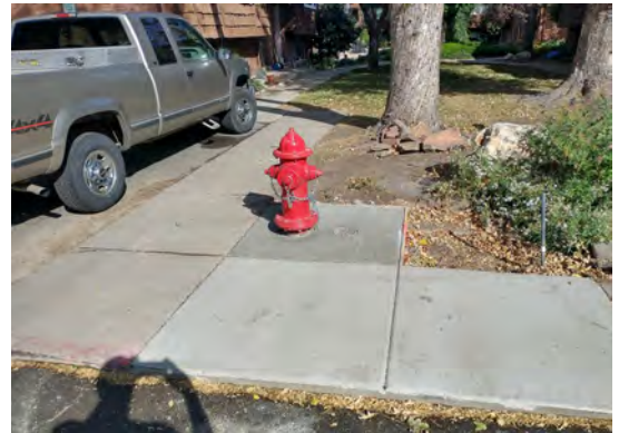
New fire hydrant pad with valve and restored landscape
