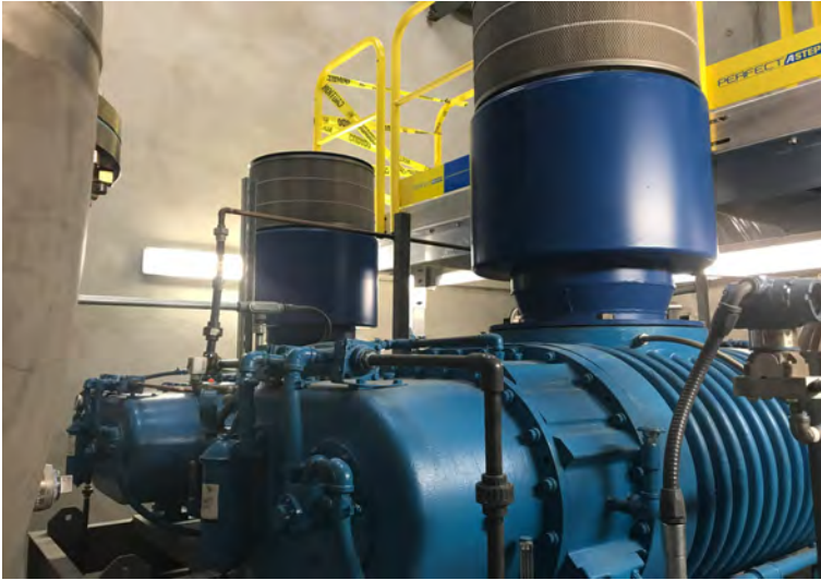
JVWTP Blower Room prior to construction
