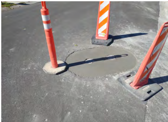
Concrete collars poured around two mainline valves in street
