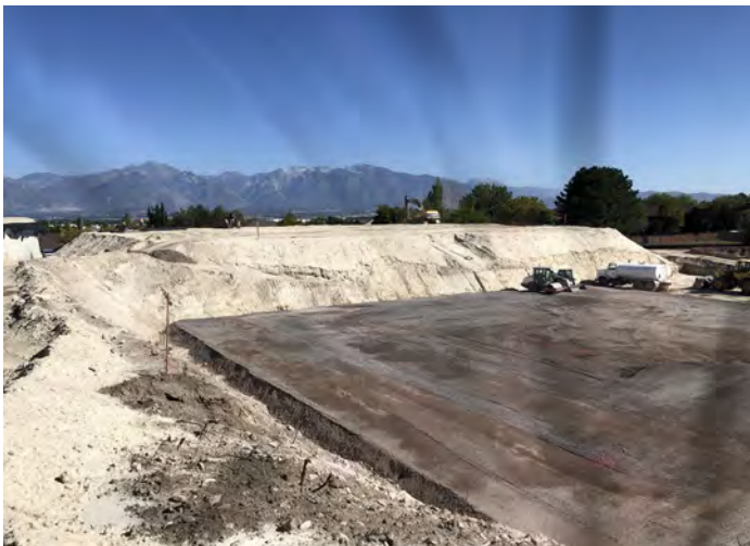
Subgrade preparation for the west side reservoir foundation
