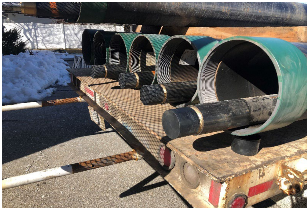
New 14-inch column pipe, tube, and shaft.
