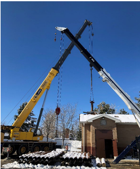
Removing pump equipment at the Newbury well.
