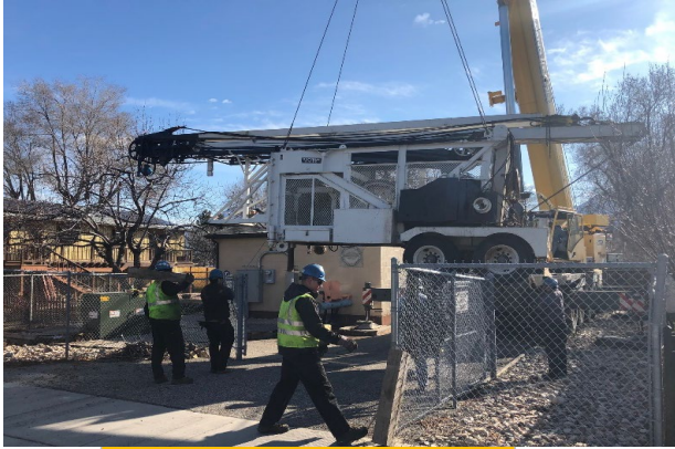
Setting development rig at the 8200 S 700 E well.
