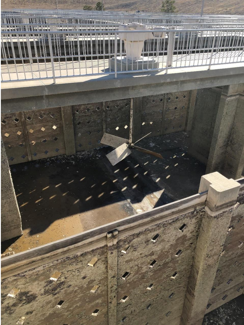
Figure 3.3 Existing Flocculator, Baffle Walls, and Stator Baffles
