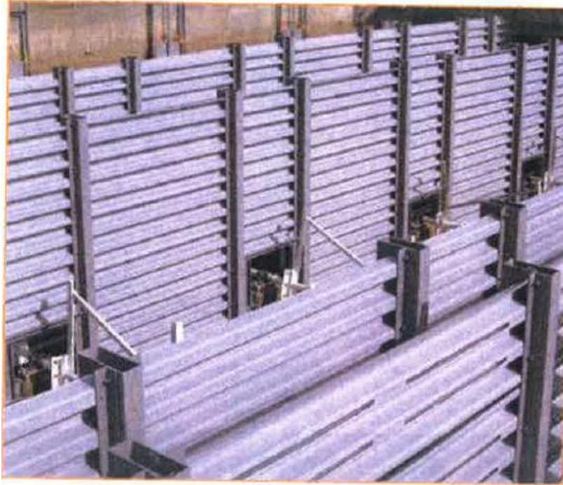
Figure 3.8 FRP Structural Baffle Wall System
