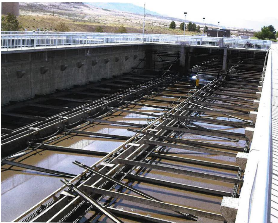
Figure 4.9 Cleaning 1985 Basins/Repairing Broken Chain and Flights
