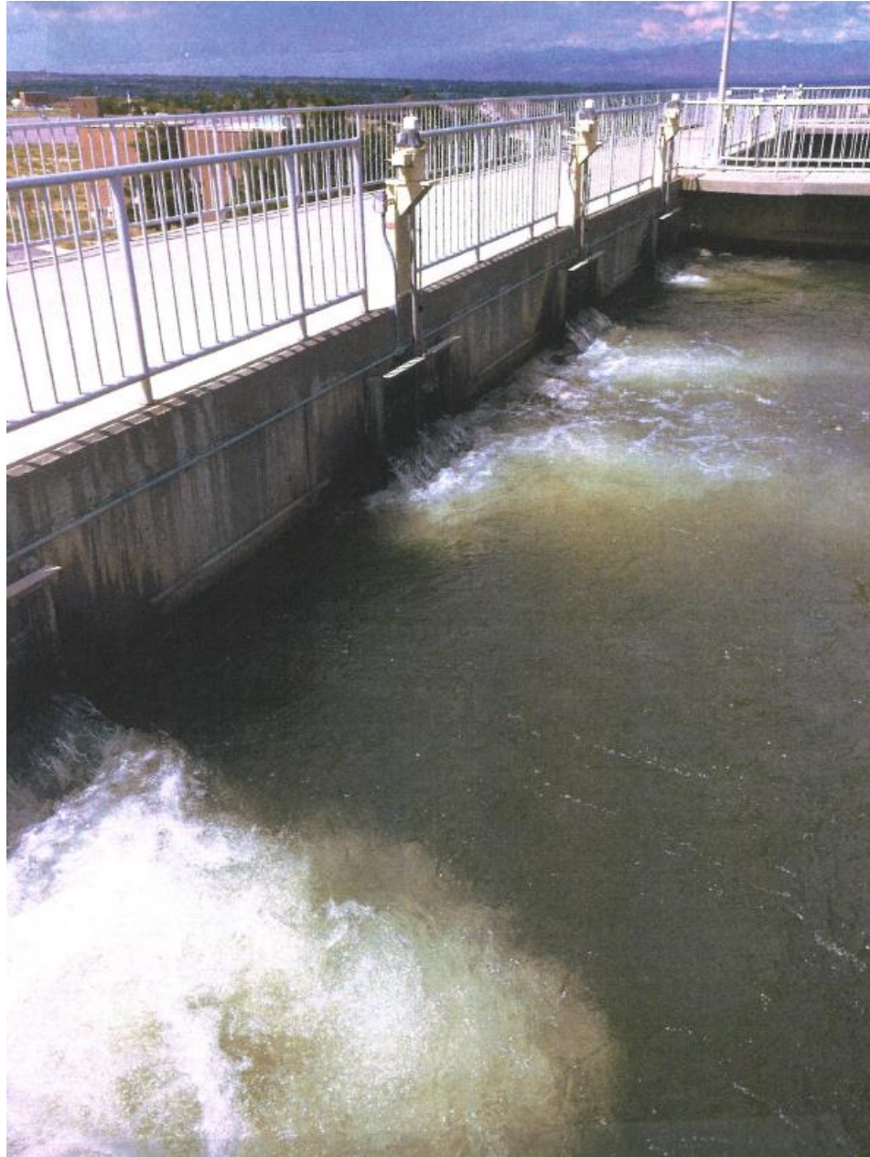
Figure 3.4 1985 Basins Slide Gates
