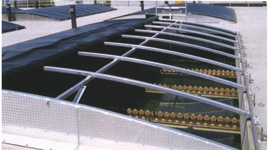
Figure 4.11 Structurally Supported Retractable Covers
