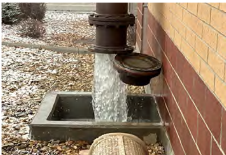
Clean water after 8 hours of pump to waste development
