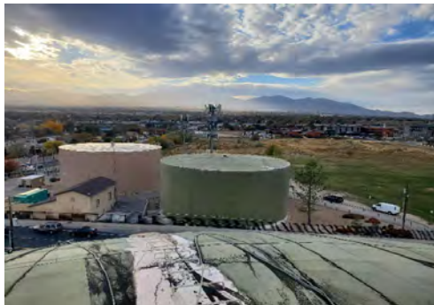
2-MG Reservoir Exterior Prime Coat
