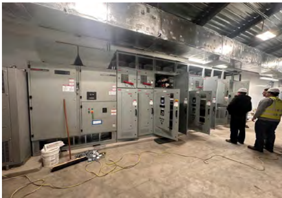
Installation of electrical equipment at 36 & 102 Pump Station
