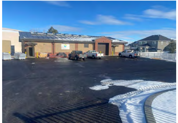
Current exterior progress of the new pump station
