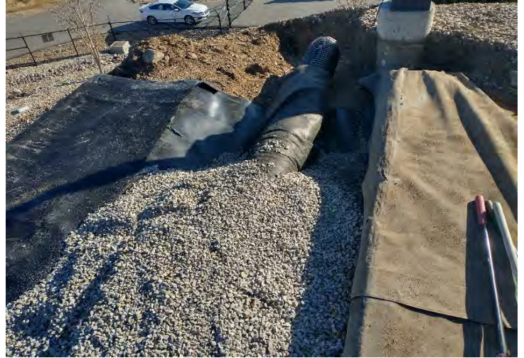
New drainage piping, wrapped in fabric, with new gravel on top
