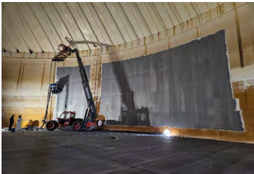
6-MG Reservoir Interior Sandblasting
