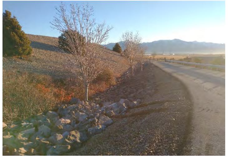
Riprap placed in channel around reservoir
