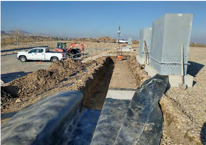
Trench on top of reservoir for new piping
