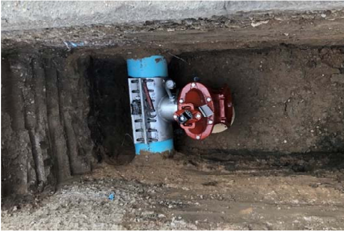
Hot tap connection to the 500 East pipeline.
