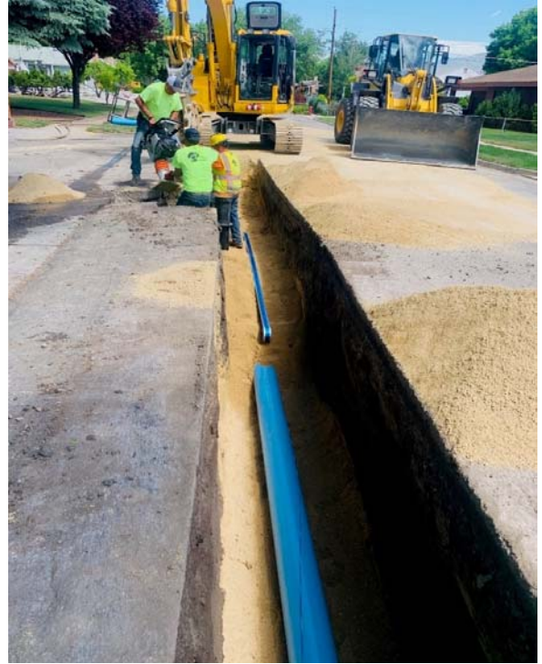
Installation of the 8" pipeline along 610 East.
