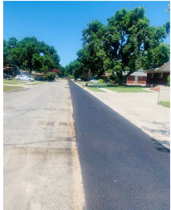
Asphalt restoration along 610 East.
