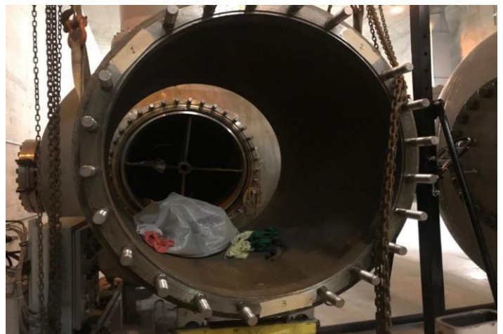
Repairs being made on JA-4 Sleeve Valve
