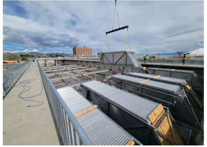
Installation of plate packs
