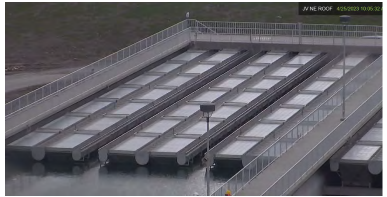
Installation of plate packs
