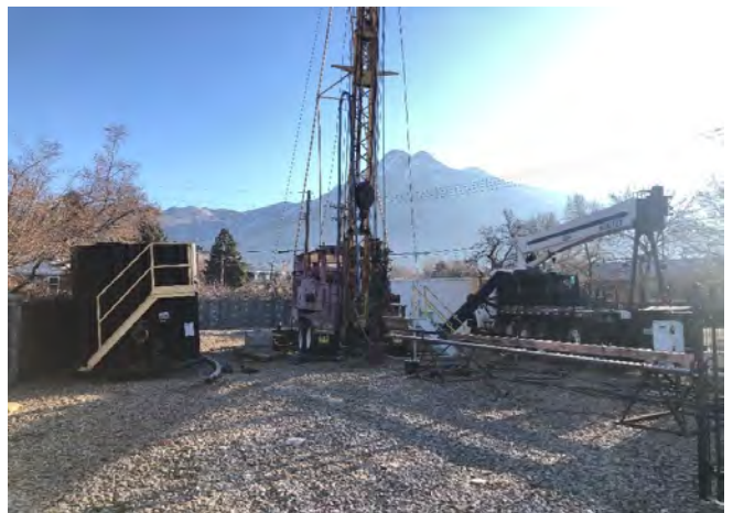
Drill rig for redevelopment of the Murray-Holladay well
