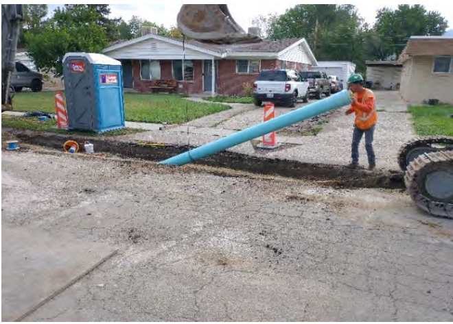
Laying new 8-inch PVC Waterline
