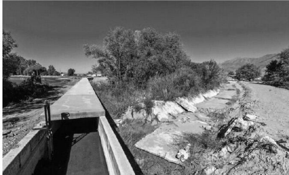
Newer, high tech canals of the Bear River Canal Co., left, are replacing older canals, right, in an effort to conserve more water and decrease evaporation.
