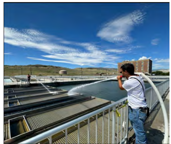
District operators washing down the plate packs
