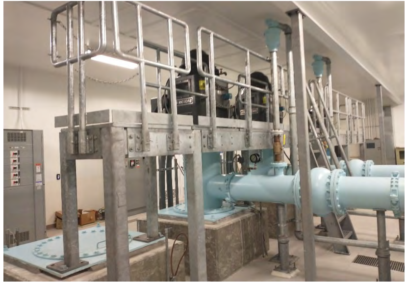
New motor access platforms
