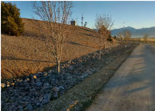
New riprap laid in channel at base of reservoir
