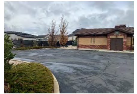
Deep Well 7 Pump Station
