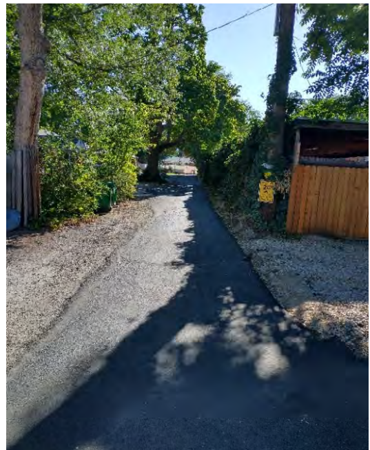
New asphalt over waterline trench
