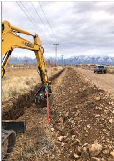
Excavation to install AC mitigation cable
