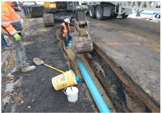
Backfilling new pipeline in trench
