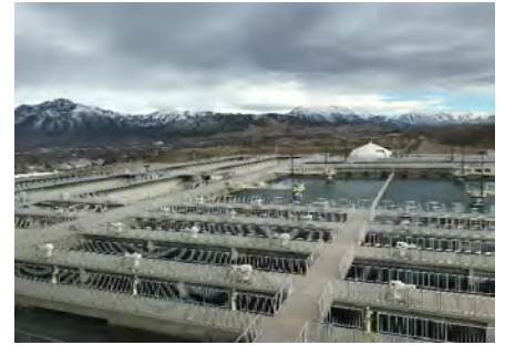
Existing Basins 1-2 in operation
