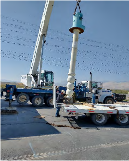
Installation of new pump
