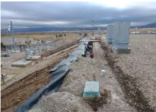
Laying drainage pipe in ditch beside top of the reservoir
