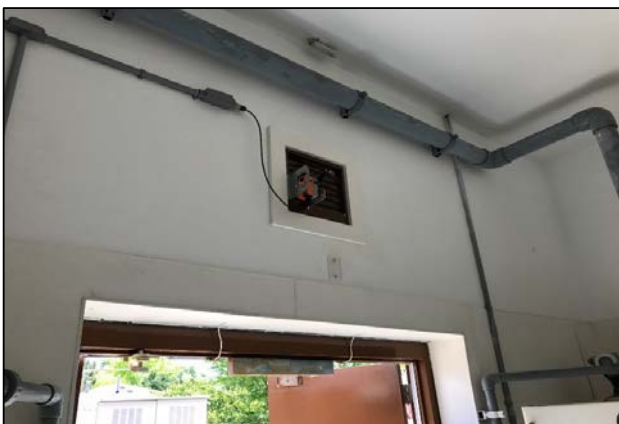
New fresh air motorized inlet louver
