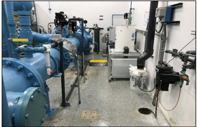
New ventilation fan at Siesta Well
