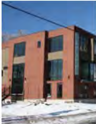
Primary Materials: Brick
