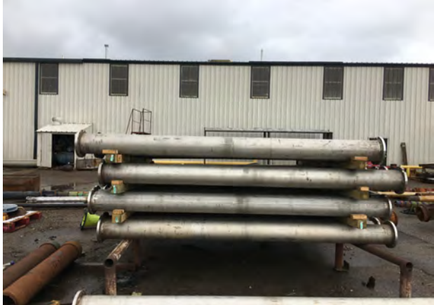
Reconfigured stainless steel well casing being reinstalled
