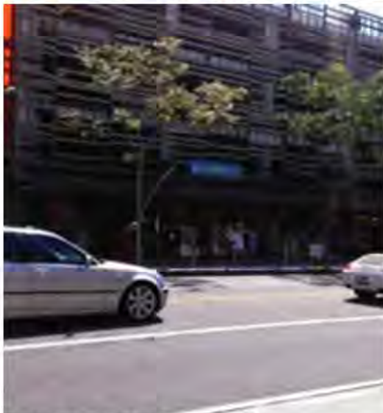
Figure 5.7 (1). Parking Structure Examples
