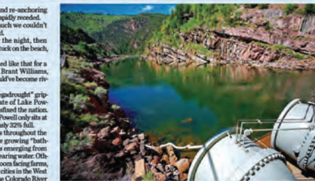
Reservoir water can be released through outlets at the base of the dam.
