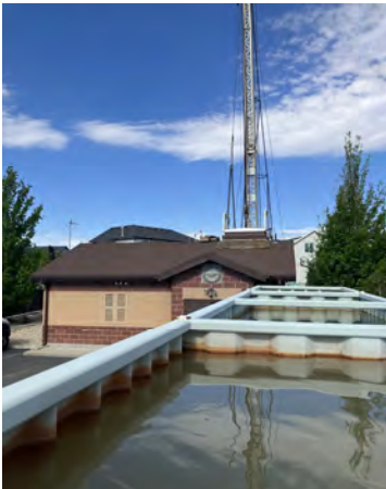
Settling tanks from well development and cleaning
