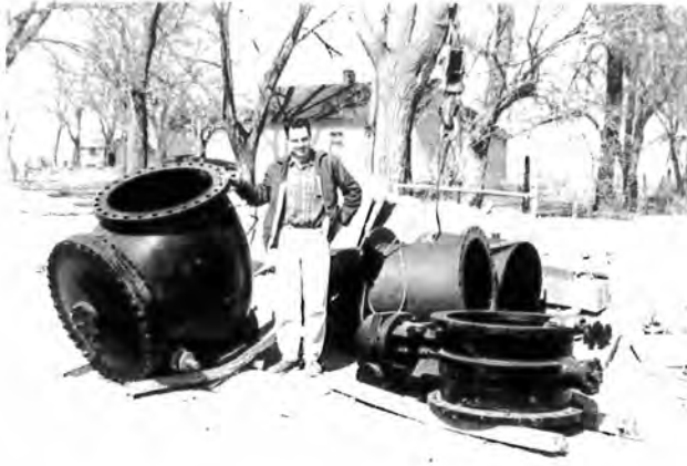
Modern pipe installation 1961
