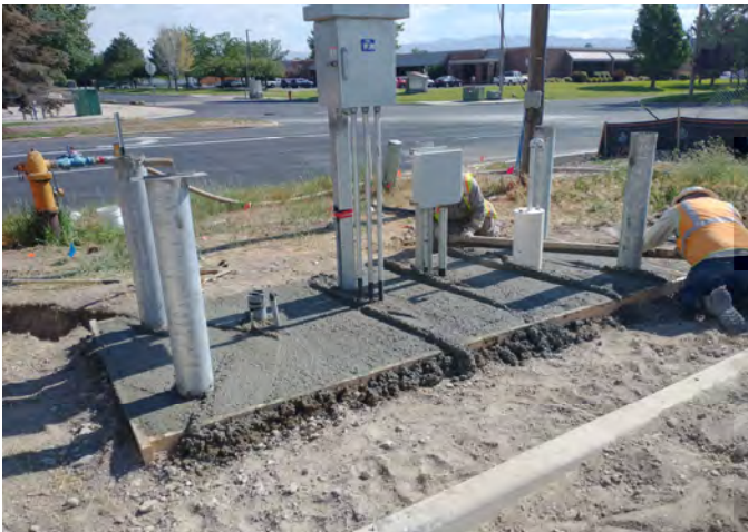
Laying concrete for new rectifier and well pad
