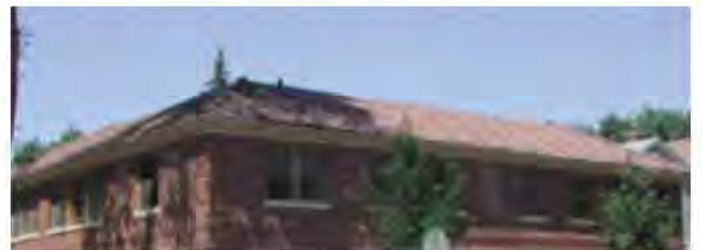
Roof Materials: Ceramic Tile
