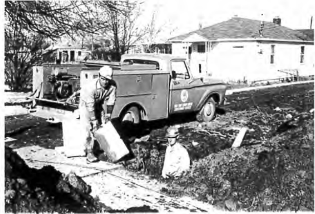
Repairing water lines 1960's
