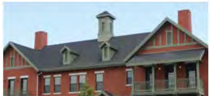
Roof Materials: Asphalt Composite Shingles
