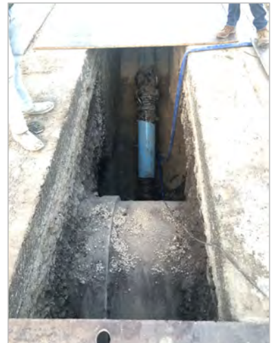
Looping waterline beneath 54" storm drain
