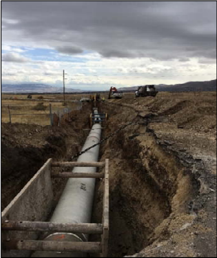
48" diameter pipe line at the intersection of 11800 South and U-111
