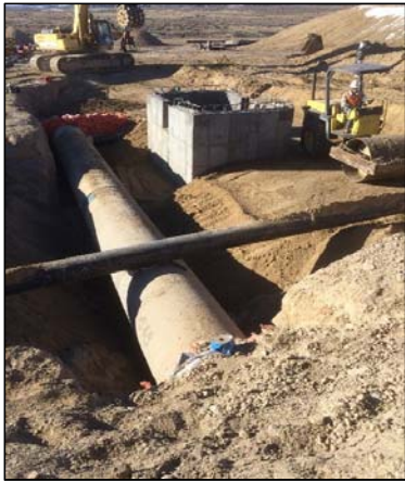
The KUCC #16 water line crossing the 48" diameter water line at the future Zone C Reservoir site
