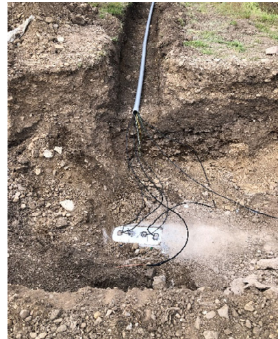
Cables cad welded to the 42" pipeline
