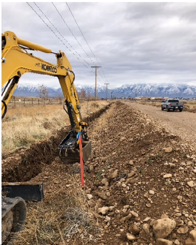
Excavation to install cable
