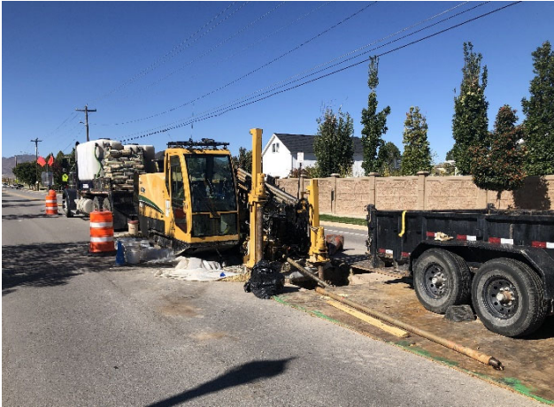
Directional drill rig
