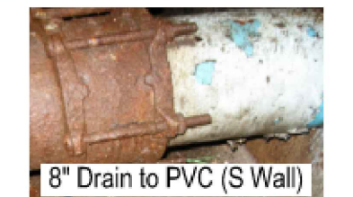
8" Drain to PVC (S Wall)
