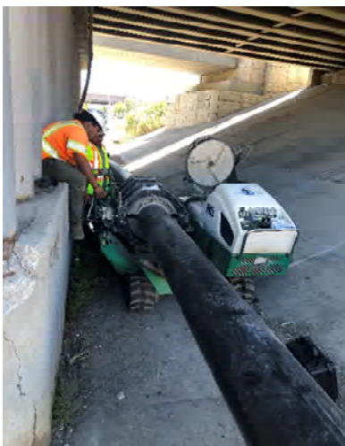
Fusing HDPE beneath 1-15 preparing for a 760-foot directional drill
