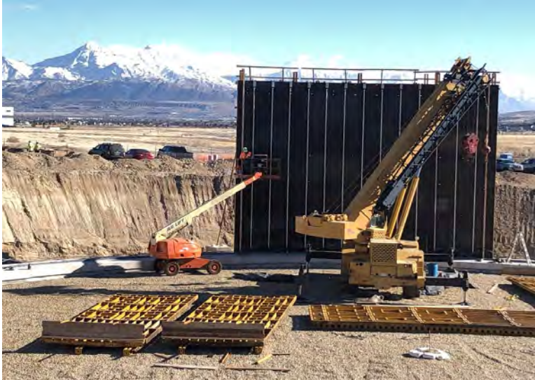
Setting first section of wall forms
