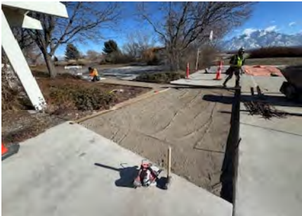
Preparing the sidewalk for concrete placement
