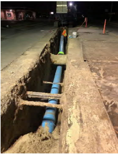
Installing 12-inch PVC pipeline
