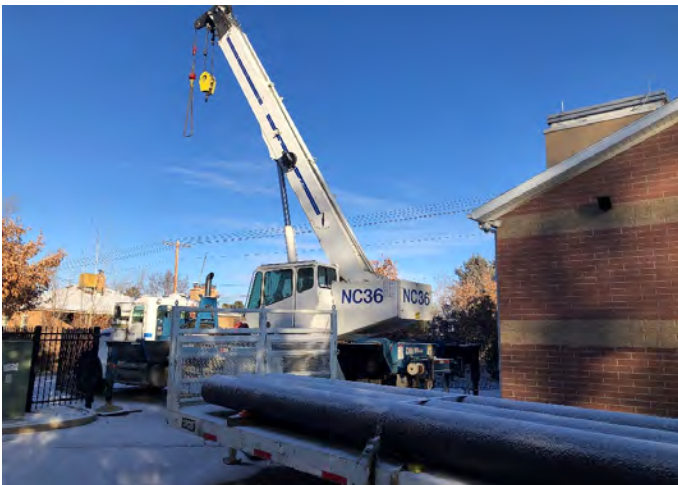
Reinstallation of the pumping equipment
