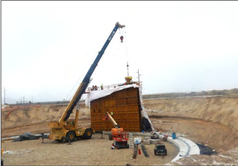
Placing concrete at top of wall
