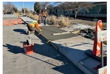
Concrete placement west sidewalk
