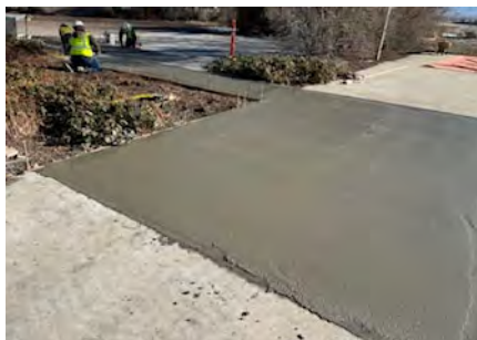
Concrete placement
