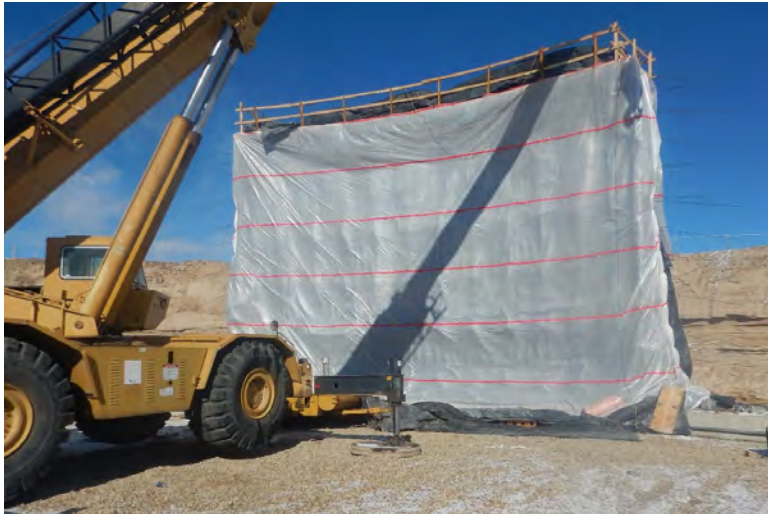
Wall segment with visqueen wrap and blankets for concrete curing
