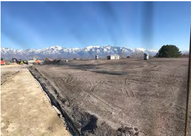
Backfill around the reservoir nearing completion
