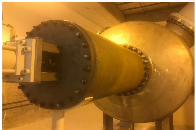
SV-2 at the JA-2 Flow Control Structure
