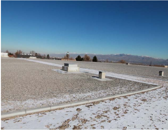
North-east view. Roof, curb and access road
