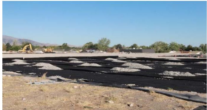
Geofabric installation
