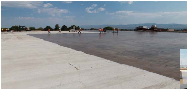
Sealant application over roof-deck Basins 1 and 2
