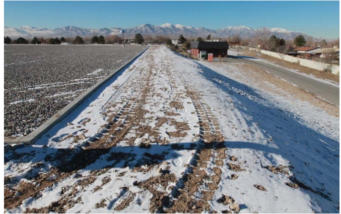
West view. Embankment, curb and roof
