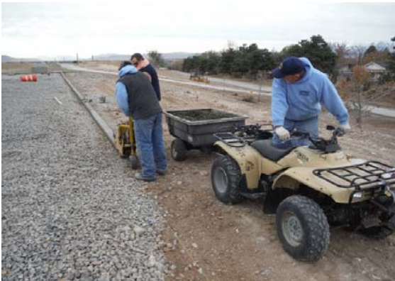
Perimeter concrete curb placement
