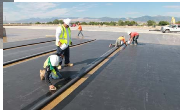
HDPE Membrane installation
