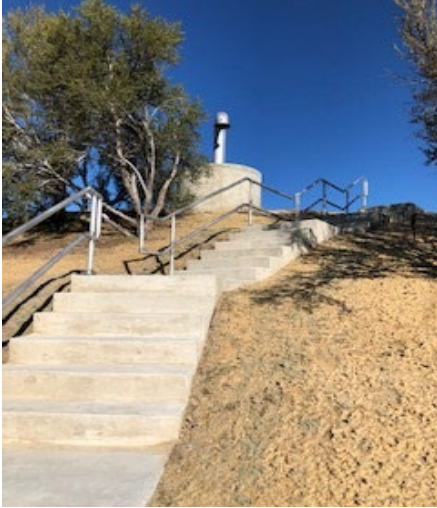
New concrete stairs at 9800 South 2300 East Reservoir
