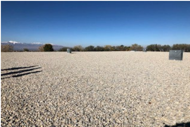
New roof deck gravel at 9800 South 2300 East Reservoir
