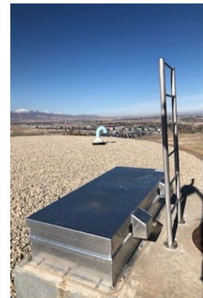
New access hatch at JWTP Culinary Reservoir
