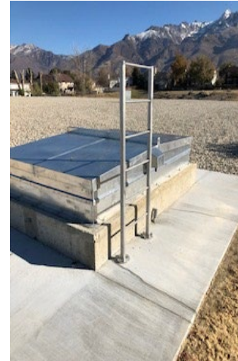
New access improvements at 9800 South 2300 East Reservoir
