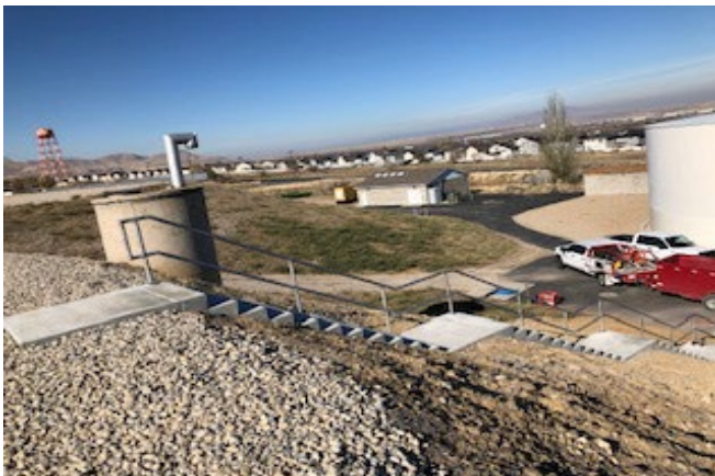
New concrete stairs at 6000 West 4700 South Reservoir
