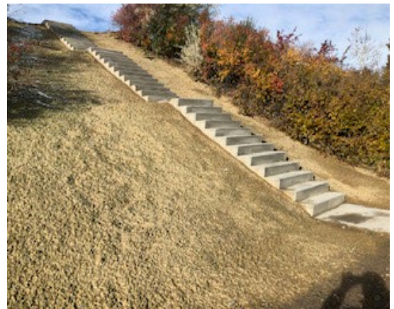
New concrete stairs at 5200 West 6200 South Reservoir
