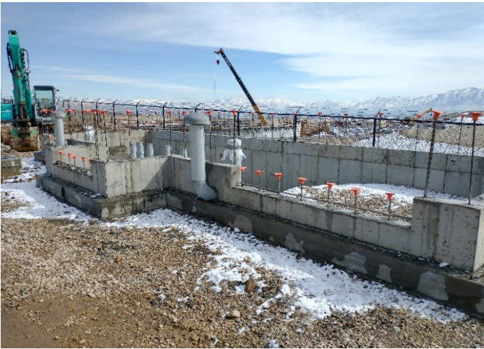
Laying walls and vents for new building
