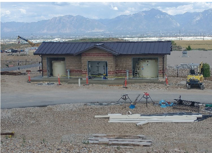
New building with roof, sidewalk, and chemical storage tanks
