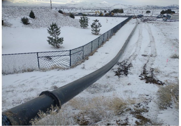
Laying new HDPE line
