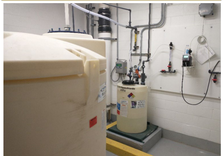
Chlorine Feed System in New Chemical Building
