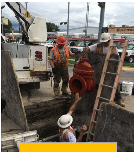
Setting 12" gate valve at 3900 South Main Street
