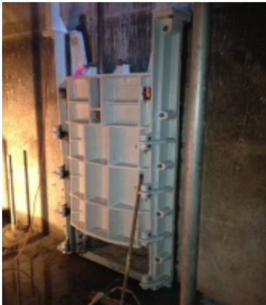
Replacement gate in flocculation basin
