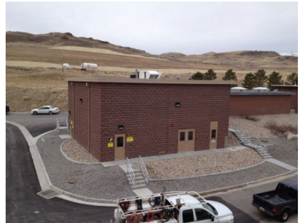
Finished Chlorine Dioxide Feed Building
