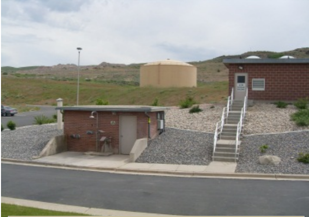
Pre-construction photo of old alum transfer
