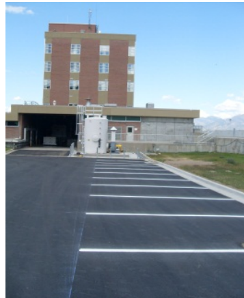
Replacement chlorine scrubber and parking improvements
