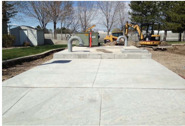
2100 South 3737 West vault
