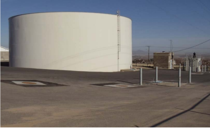
4700 South 6000 West Reservoir site
