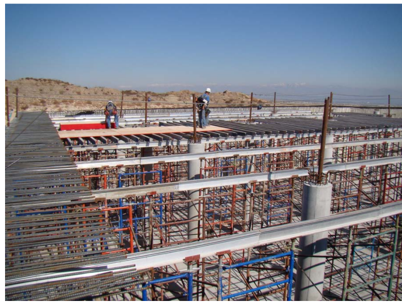
Construction of the reservoir deck.
