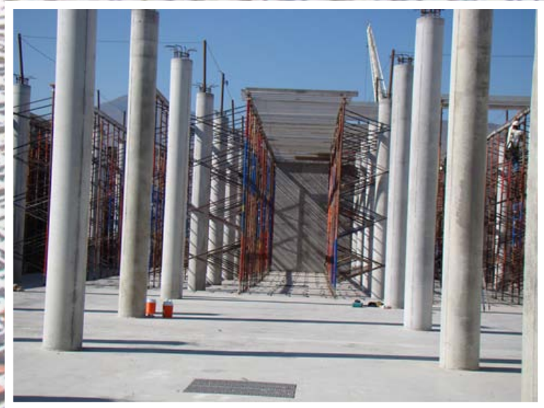
Scaffolding for reservoir deck.
