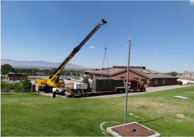
Delivery of Generator
