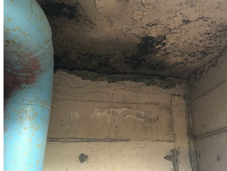
FAILING CONCRETE WALL
