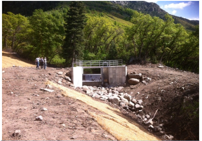
Completed Middle Fork of Dry Creek Diversion Structure
