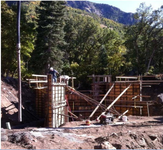
Construction of the Middle Fork of Dry Creek Diversion
