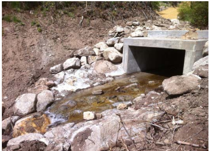
Middle Fork Stream Restoration Structure
