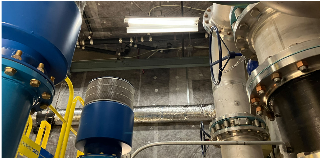
4" of sound attenuating foam on walls
