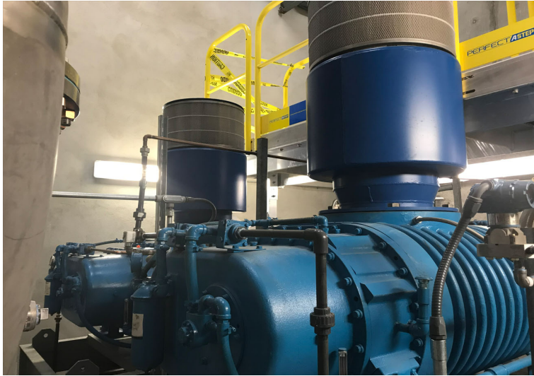
JVWTP Blower Room prior to construction
