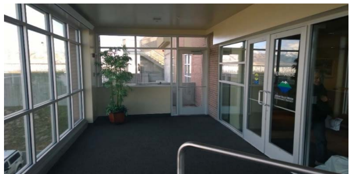
New lobby interior and existing entrance
