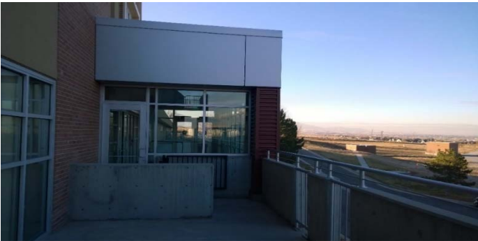
New lobby west view
