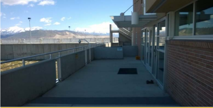
View of previous access to the Laboratory and High-rise
