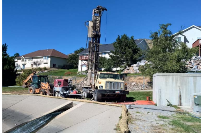
Drilling anode well at Lindon Reservoir Site
