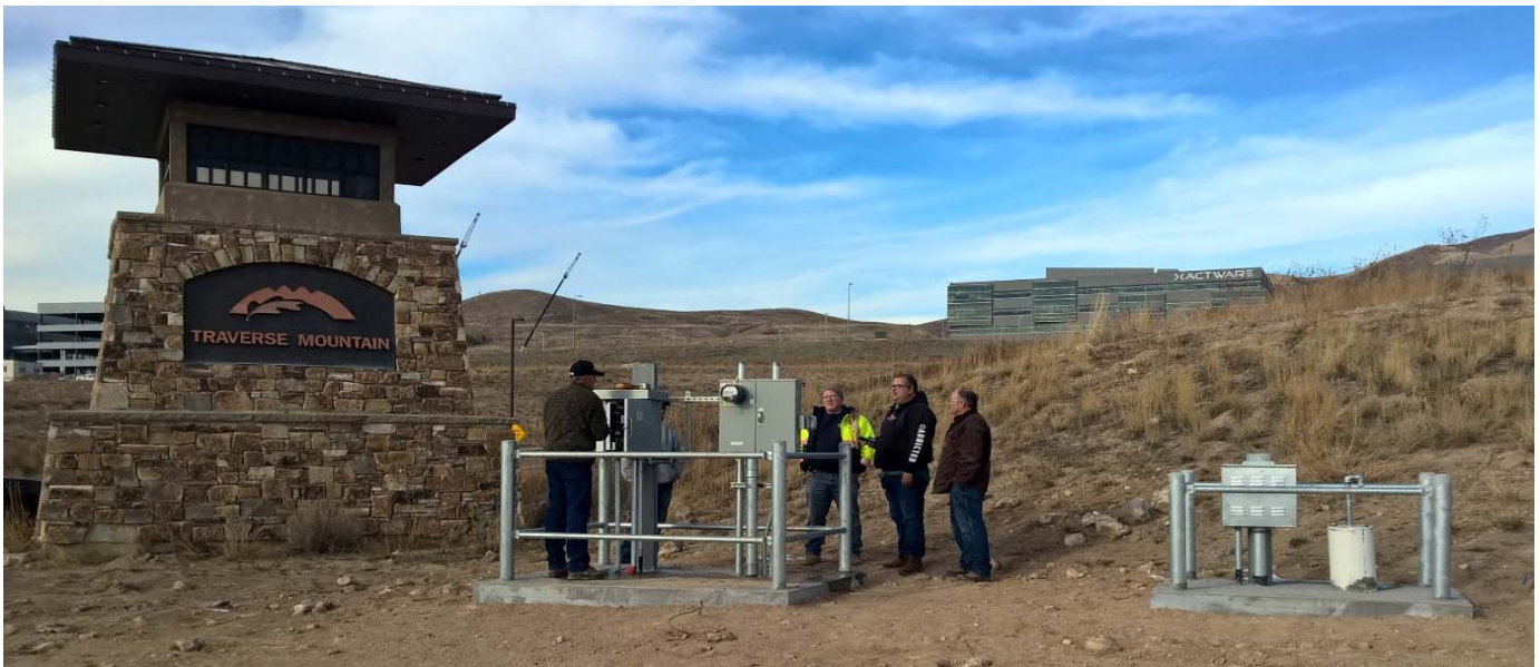
Completed installation at Morning Vista Road
