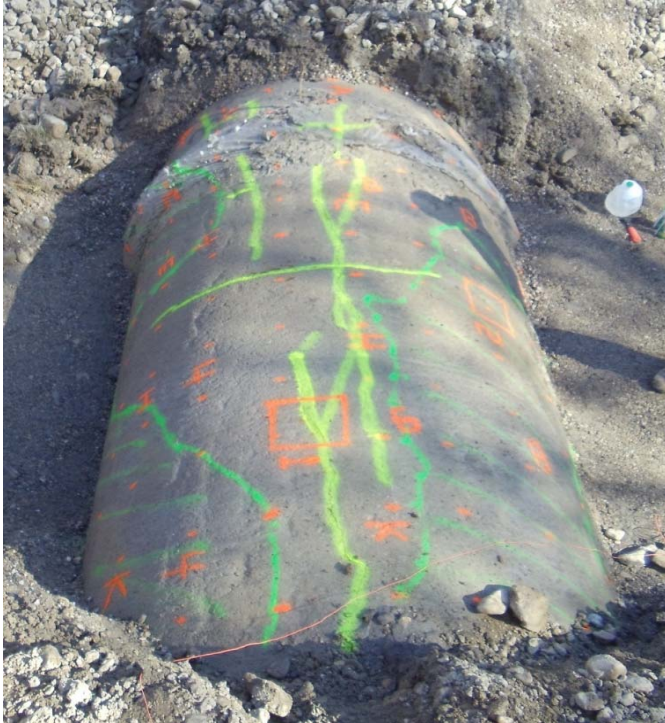
Assessing condition of the Jordan Aqueduct
