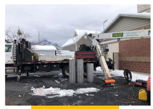
Staging equipment to install well swage
