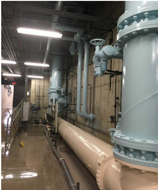
New basement floor protective coating
