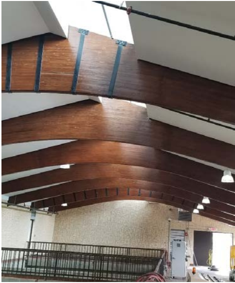
Repaired coated glulam beams
