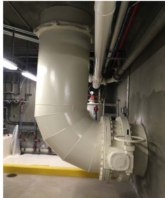
Filter gallery pipe recoating
