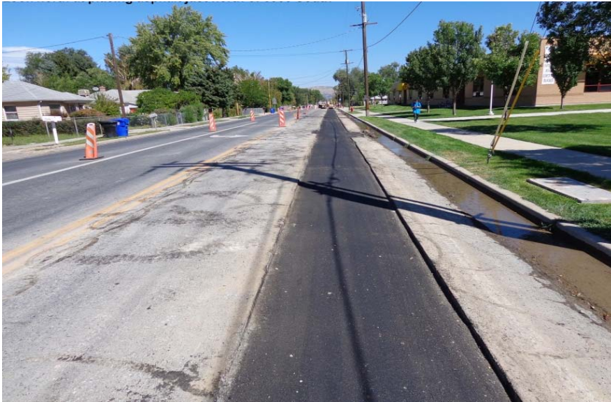
Asphalt Paving on 500 East
