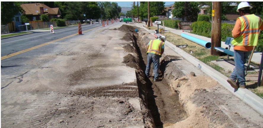
Compacting backfill on 500 East
