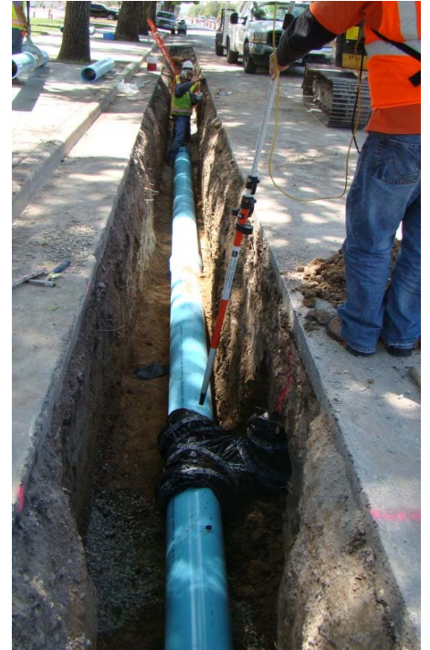
GPS locating of fittings on 500 East Pipeline
