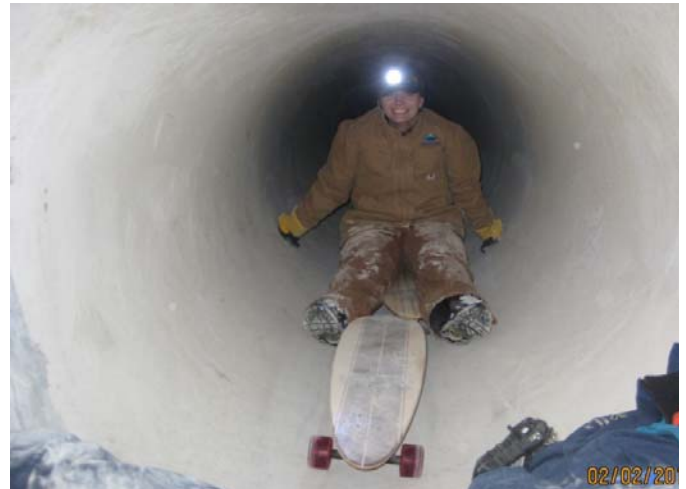
Pipeling inspection by District staff
