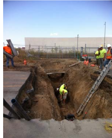
Connection to West Jordan City at Dead Man's Curve
