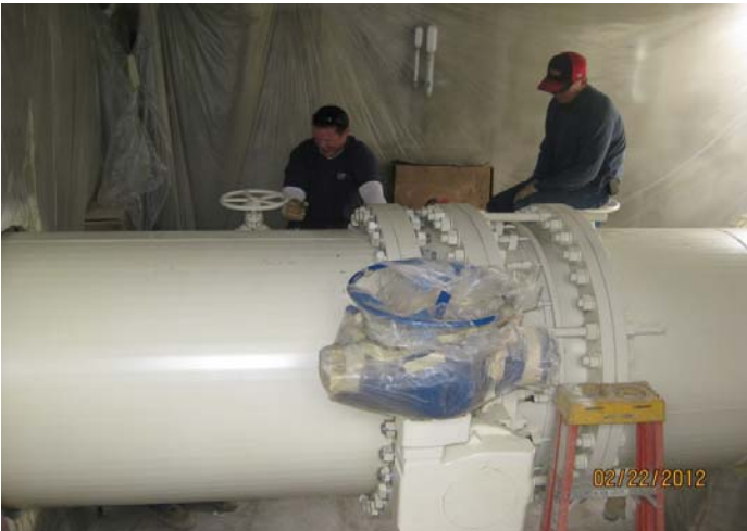
Painting inside a mainline valve vault
