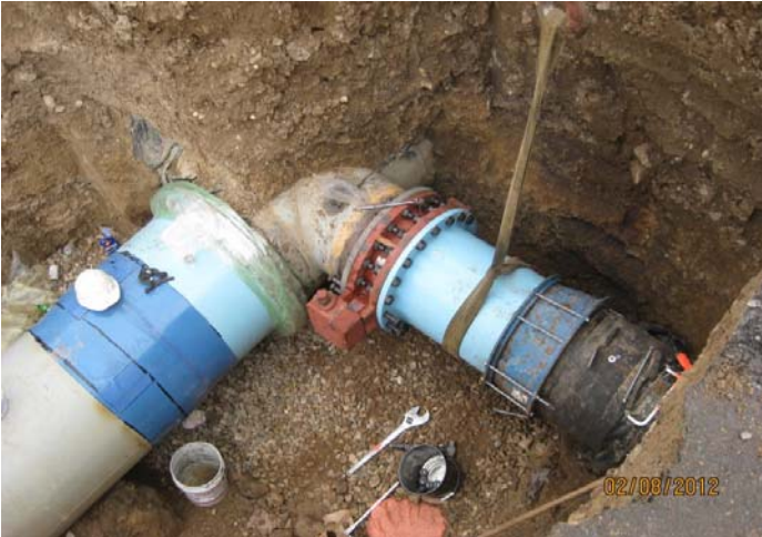
Connection to the new pipeline at the Zone D
