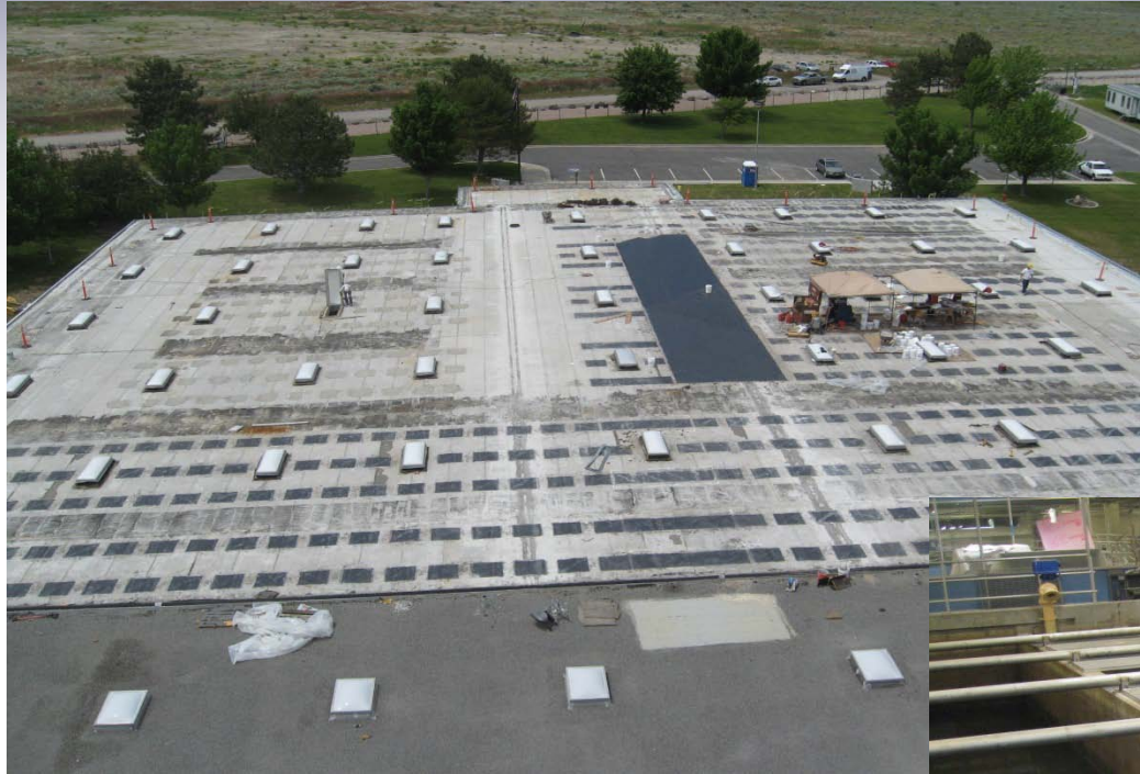
View of the building's roof FRP installation
