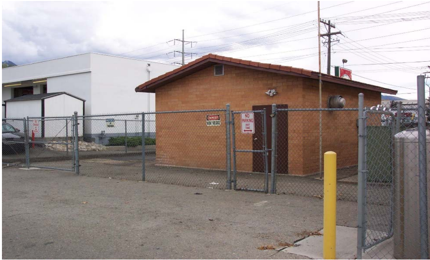
1300 East 7000 South Well House
