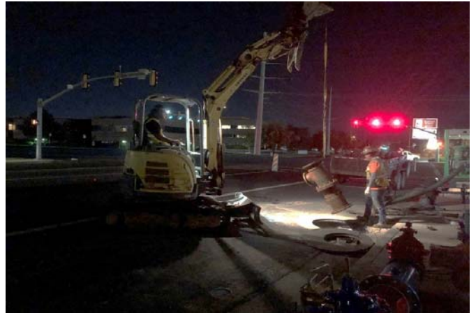
Removal of existing vault piping.
