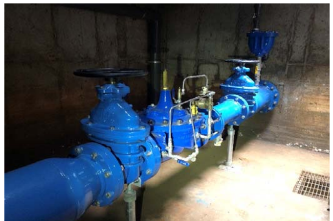
New vault piping and valves.
