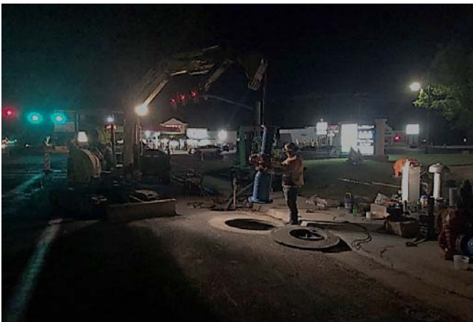
Lowering new piping into vault.
