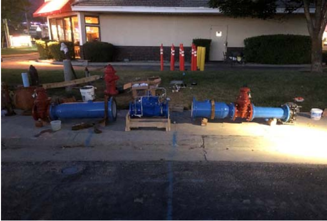
Staging material for night time water shutdown to minimize customer impact.
